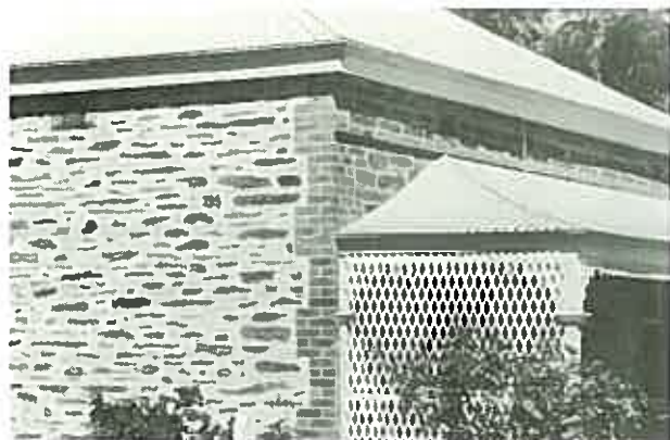
A sophisticated house of random rubble which is coursed and the front facade pointed. The corners and apertures of the house are trimmed in brick. (Cottage, Dundas Street, Gawler, South Australia.)
