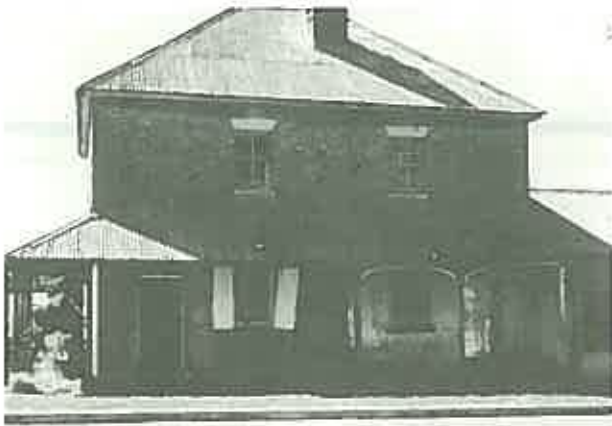
In this example of a face brick building where a small section under the verandah has been painted, paint removal can perhaps be justified. (37-39 North Street, Windsor, N.S.W. prior to restoration.)
