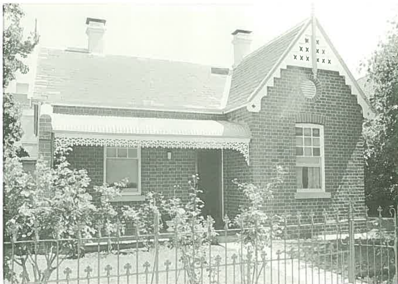
Most Edwardian brick buildings have their front wall tuckpointed. ( Verger's Cottage, St. John's, Parramatta. )
