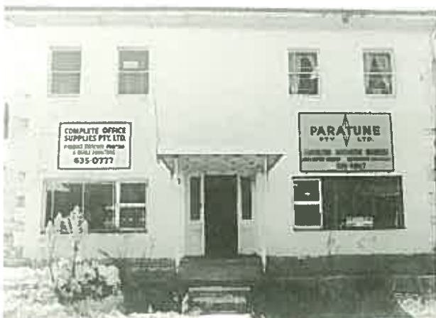
Hidden by 1950s cement render this 1820s house is unrecognisable. ( Harrisford, 182 George Street, Parramatta. )
