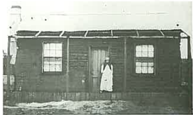
An 1870s photo of a wattle & daub cottage at Hill End, N.S.W. ( Hollermann photograph. )
