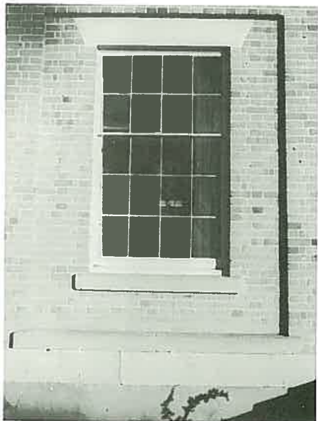
The combination of brick and stonework is an important characteristic of many colonial buildings. ( Forcett House, Fawcett, Tasmania, 1830s. )
