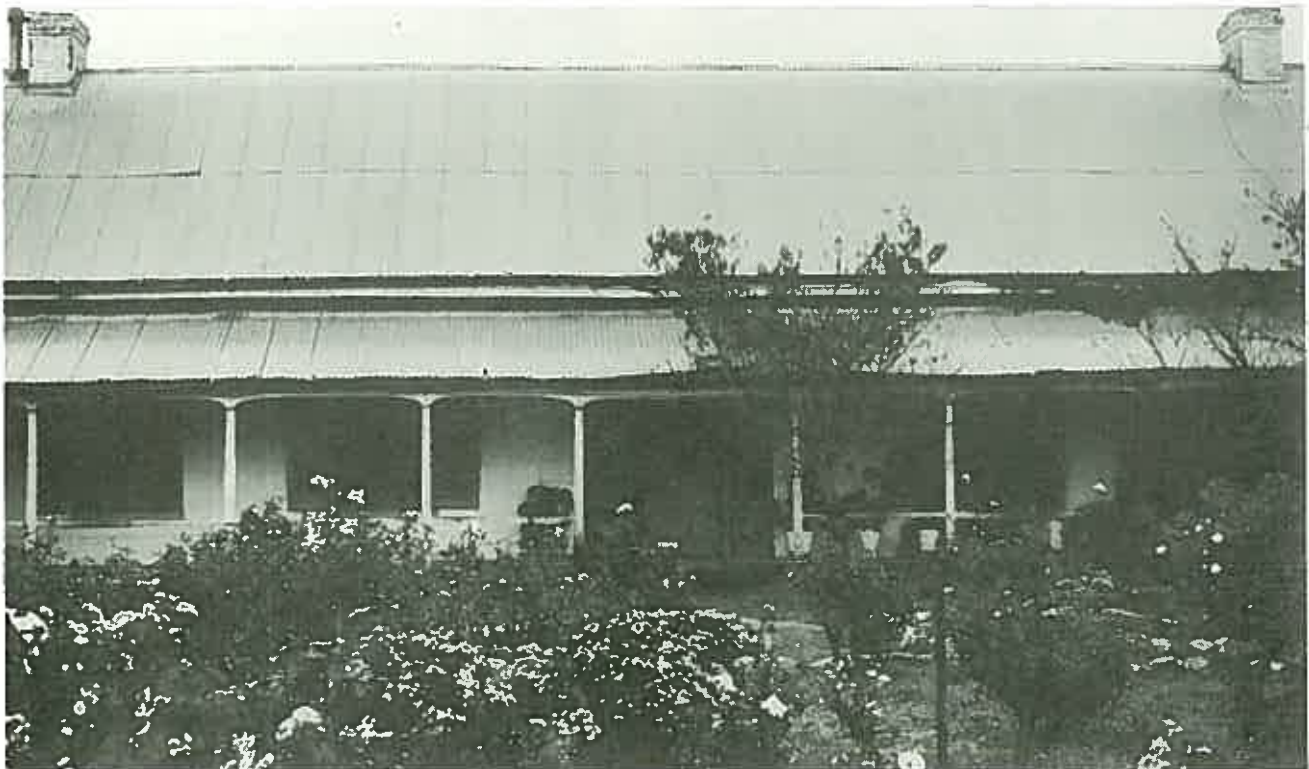
Quite substantial buildings were built of Pisé. The only way to tell is if the render is off. ( Cunningham Plains, Harden, N.S.W., 1862. )
