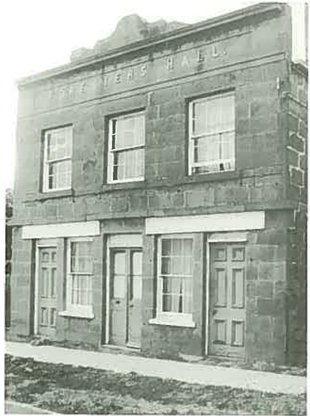
Typical of the 19th century, the dressed stone is reserved for the front wall. ( Foresters Hall, 18-20 Sackville Street, Portland, Victoria. )
