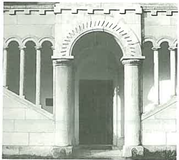
The contrast of stone tooling is part of the character of this fine building. ( St. Mark's, Pontville, Tasmania. )
