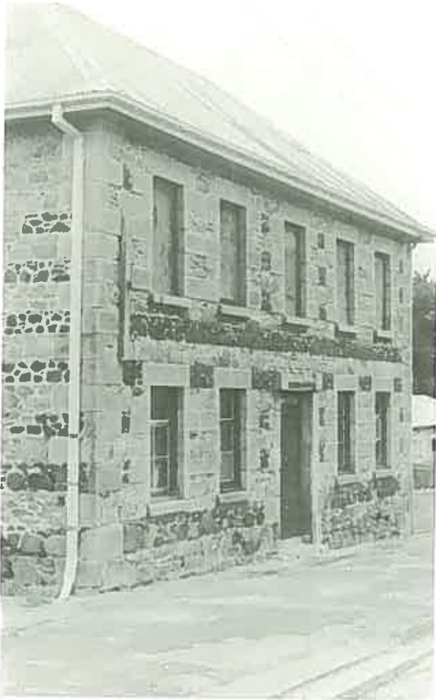
A highly individual treatment of rubble used with freestone trimming. ( Parish Hall, Avoca, Tasmania. )
