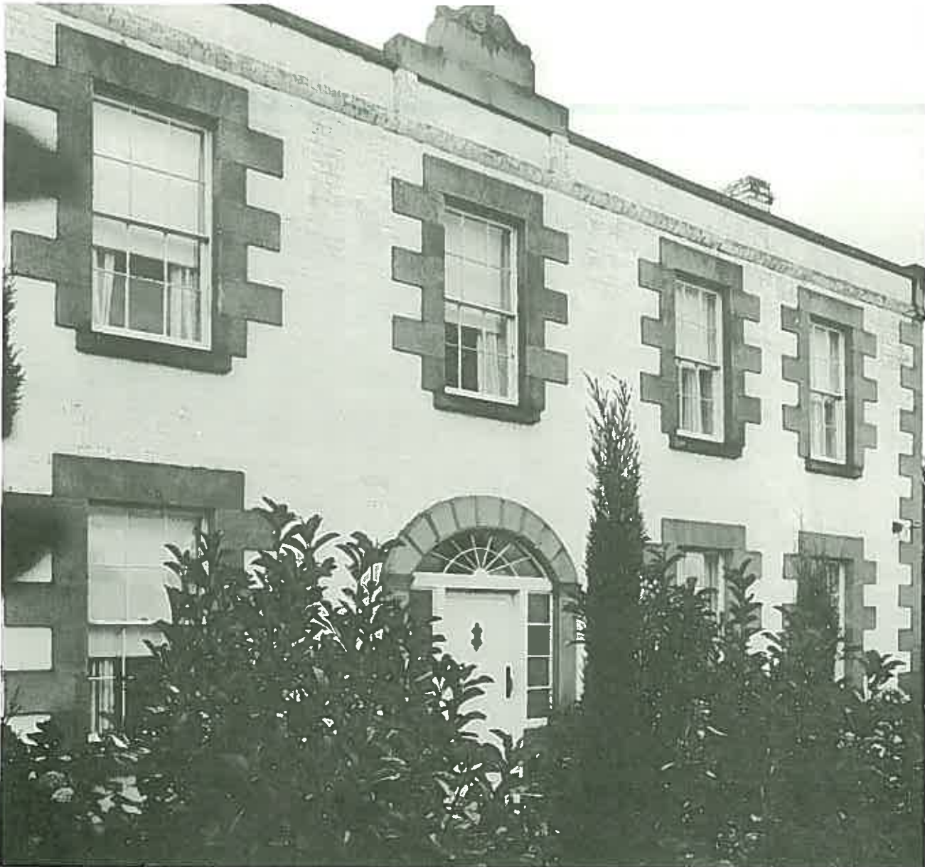
A house which combines both brick and stone in its construction to achieve a decorative effect. ( The Manor, Baschus Marsh, Victoria, c. 1840. Photo: Wesley Stacey. )
