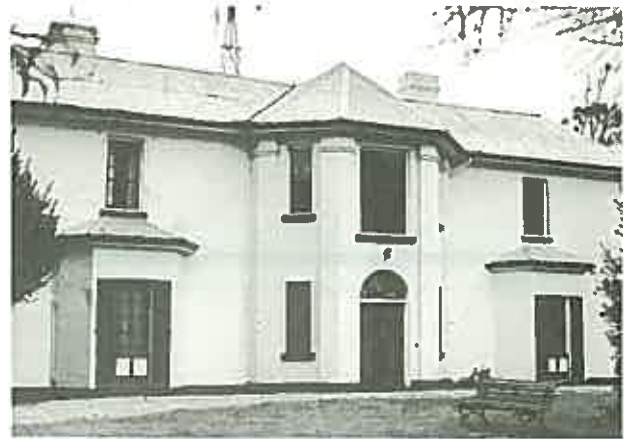
This house may well have been facebrick when it was new but it has been painted a long time, probably as much for keeping its solid walls dry as for fashion. It should continue to be painted. ( Rhodes, South Esk River, Tasmania. )
