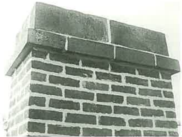
In parapets and chimneys a small amount of cement can be used to allow for more severe weathering. (Harper's House, Berrima, N.S.W.)
