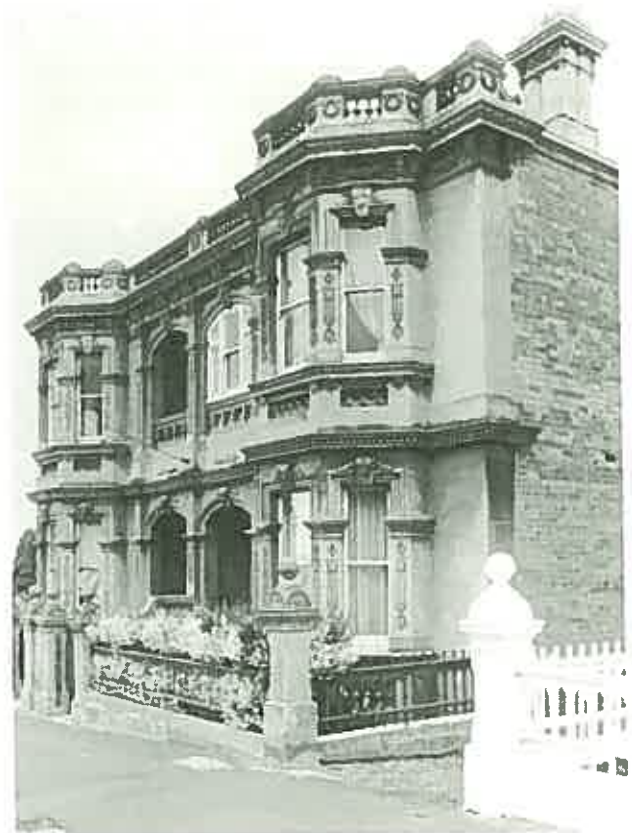
Cement became appreciated for itself and in many late Victorian buildings was left unpainted. (6-8 Church Street, Hobart.)
