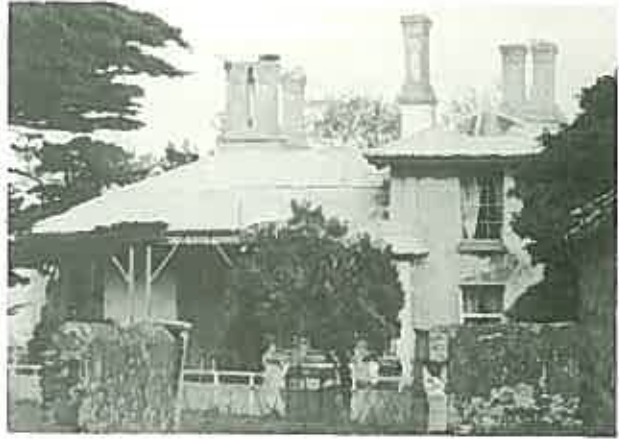
The chimneys on this 1830s house are rendered in an early patented cement. ( Highfield, Stanley, Tasmania. )
