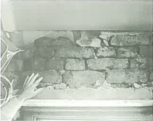
Adobe bricks used in the construction of an 1830s house near Orange, N.S.W. ( Bookanan, Byng. )
