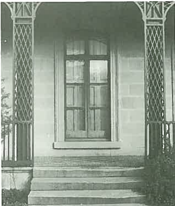
These gently worn steps are original to the house and therefore precious. ( Runnymede, New Town, Hobart. )
