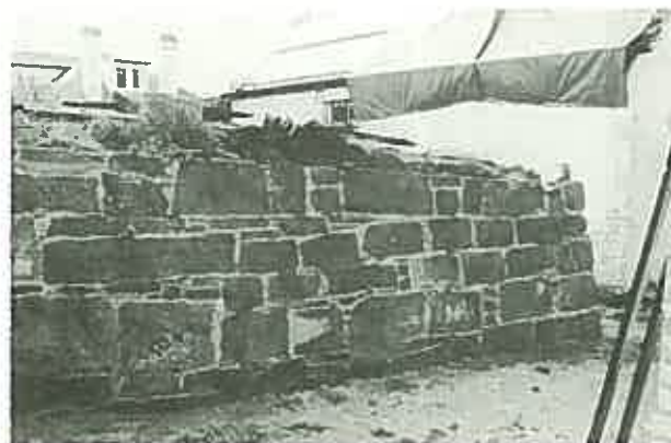
The individuality of stone walling must be appreciated as in this restored retaining wall at Port Arthur. (Priest's House, Port Arthur. Restoration architect: Clive Lucas.)
