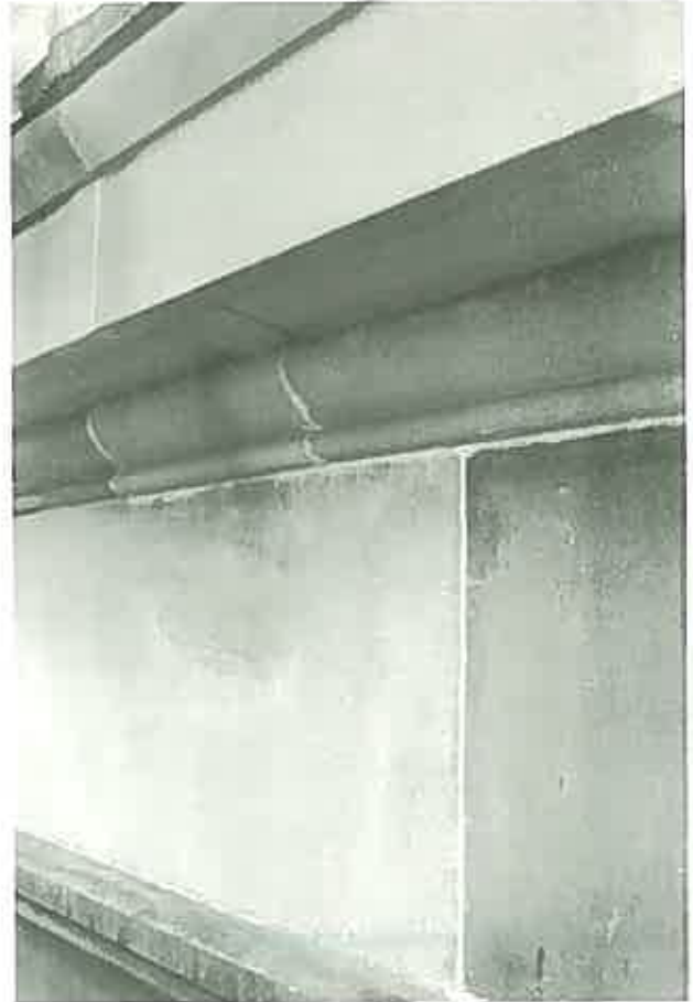
In finely rubbed work a mason's putty joint is usually employed. ( Pitt Street Parish Church, Sydney. )
