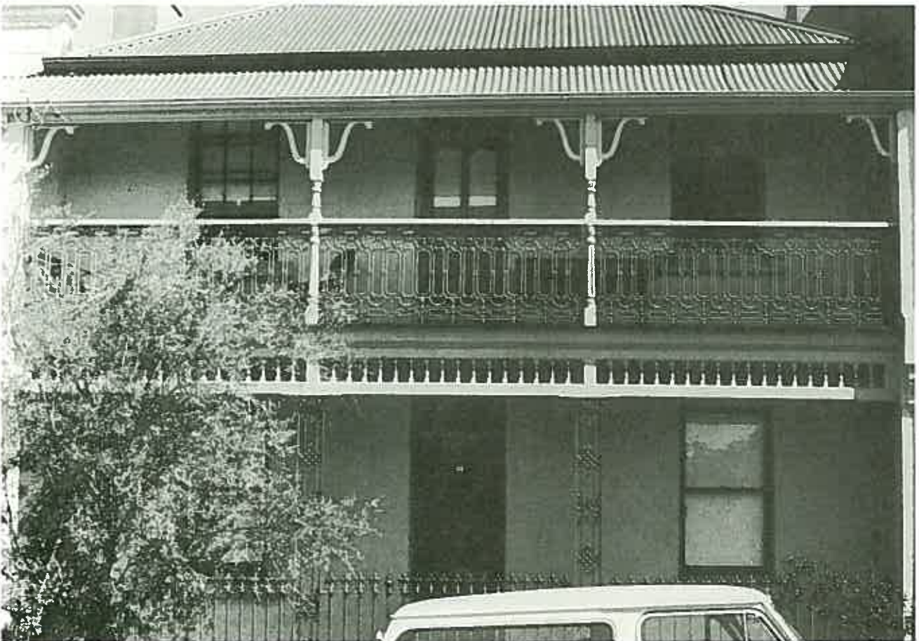
In this Sydney example the rendering has been put back, not only restoring the correct character to the house, but also making it considerably more waterproof. (Restoration architect: Clive Lucas, Photo: Jyoti Somerville.)
