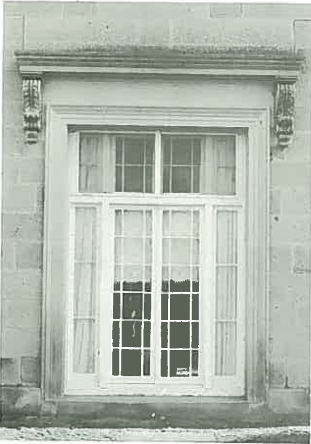
Sparrow picked ashlar with rubbed dressings produces a delightful effect. ( Wentworth House, Bothwell, Tasmania. )
