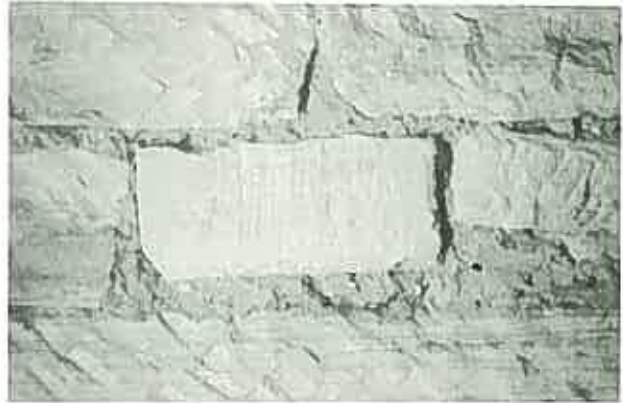
An example of shell lime mortar. Pieces of shell can actually be seen. ( Vaucluse House, Sydney. )
