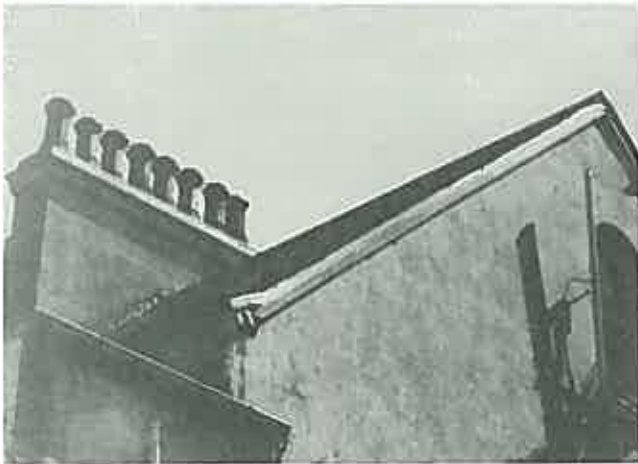
Chimneys and terra cotta pots are important features of many 19th century roofs. (43 Arundel Street, Glebe, Sydney)
