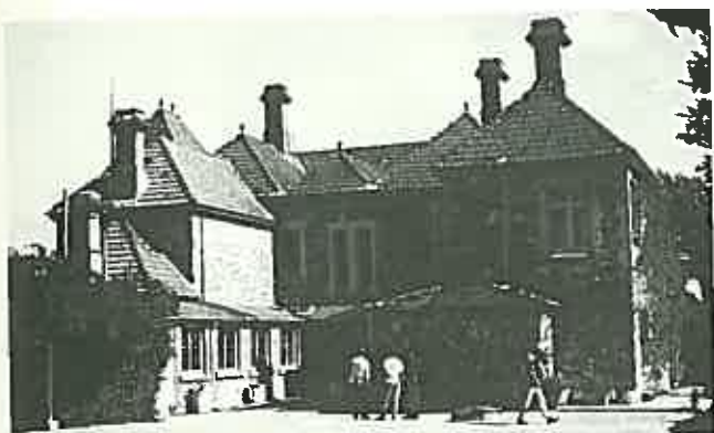
This house built in the 1870's originally had a roof of shingles but after a fire in the early 1890's it was resheeted with the newly available French Marseilles patterned tiles. (Currendooley, Bungendore, N.S.W.)
