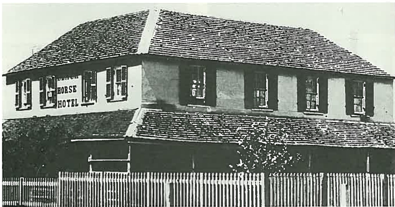
Nineteenth century photograph of Black Horse Inn, Richmond, N.S.W. with shingled roof and iron ridging. (Photo in possession of Hawkesbury Agricultural College)
