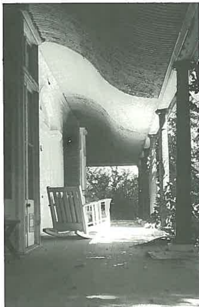
When iron was curved it needed little support as shown in this verandah. (Hartwell House, Kiama, N.S.W.)
