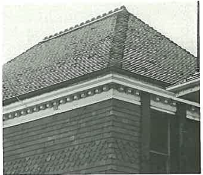
Flat terra cotta tiles were popular for roofs and also walls of Queen Anne style houses. Here there are matching hip and corner tiles, cresting and shaped tiles, all of which were made in England by Burton & Sons of Staffordshire in 1887. (Caerleon, 15 Girahgulla Road, Bellevue Hill, Sydney)
