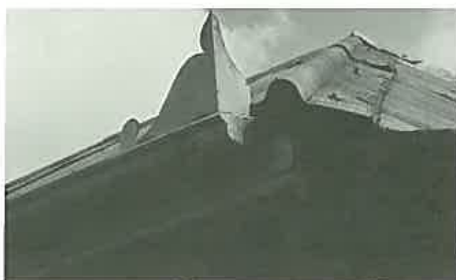
Acroterion fixed at the end of a half round gutter. Intact detail like this is very important. (Cottage, Ayers Street, Burra, S.A.)
