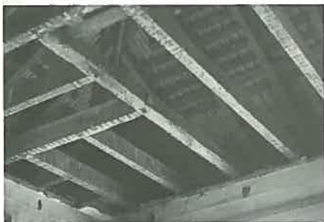
Sometimes shingles were stripped before the iron was fixed. Here shingle battens survive from the earlier roofing. (Glenalvon, Campbelltown, N.S.W. Restoration Architects: Fisher Lucas)
