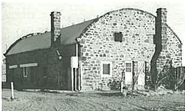
A semicircular roof has been made of rivetted curved sheets obviating the necessity for timber framing in a region where timber was scarce and transport difficult. (Station Store, Murnpeowie, South Australia. Photo: Stephen Gilbert)
