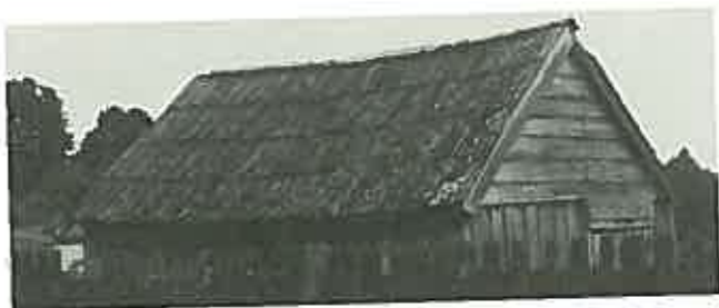
Split shingles are found in various widths and lengths. Long shingles on a Tasmanian outbuilding. (Shed, Grigg Street, Deloraine, Tasmania)
