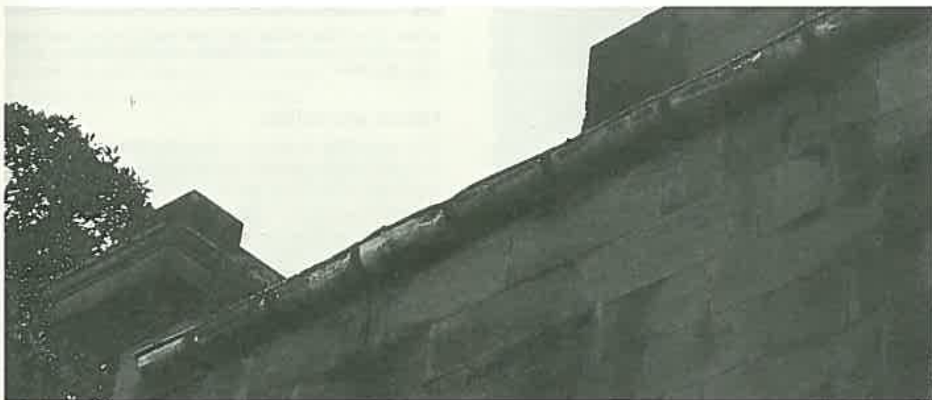
An unusual survival, a half round lead gutter on iron brackets.
