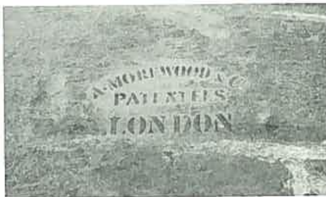
The trade label of A. Morewood & Co. patentees, London, found on the underside of the earliest iron tiles. (Kleusendorffes Inn, Tahmoor, N.S.W.)
