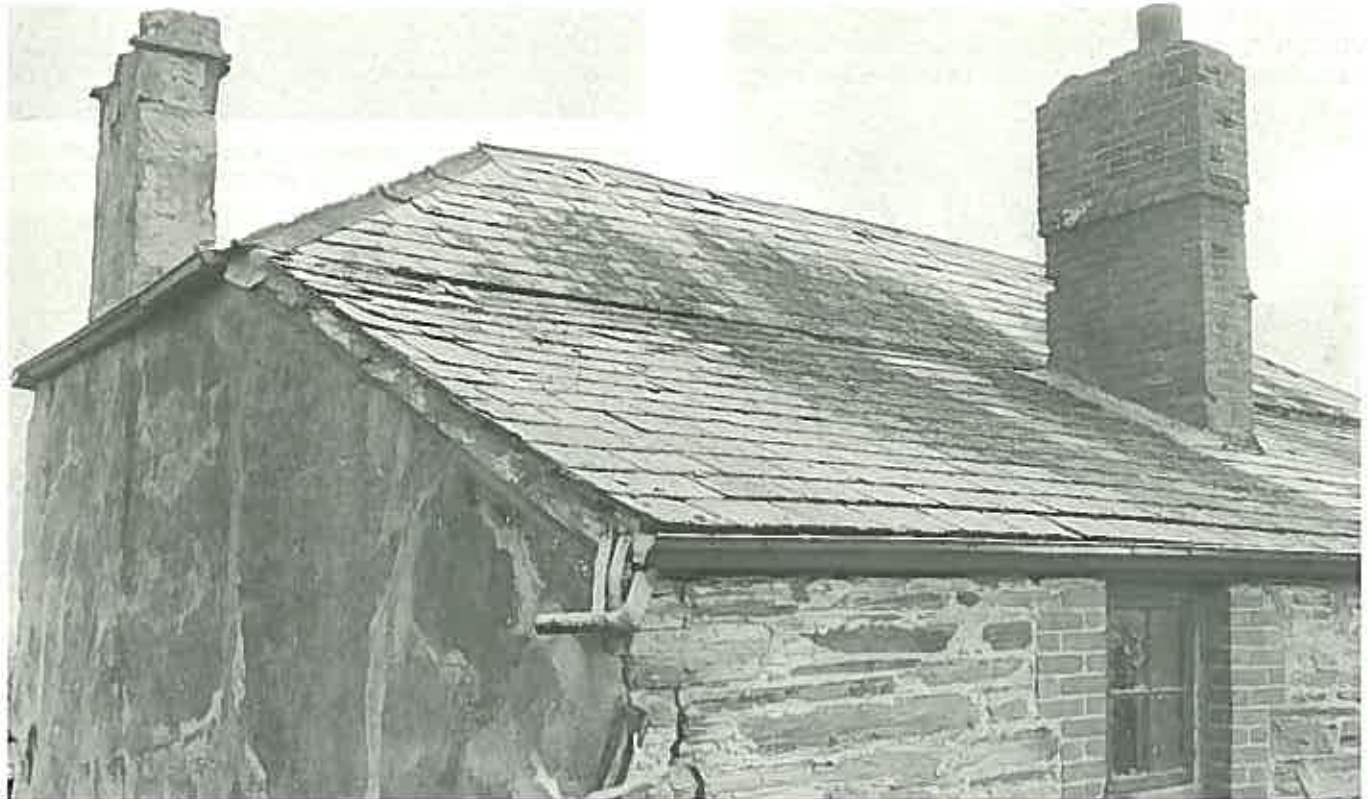
In this dilapidated example can be seen the end of the roof, the overlap of the slates and the ends of the battens. The slates were quarried within a mile of this house at Delabo Quarries, opened in 1840. (House, George Street, Willunga, S.A. Photo: Stephen Gilbert)
