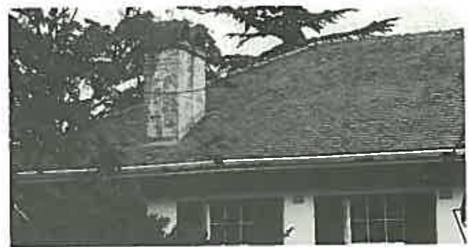
Flat tiles continued in use into this century here with half round terra cotta tile ridging. (Purulia built in 1916 and 16 Fox Valley Road, Wahroonga, Sydney)
