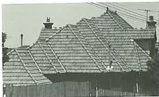
Marseilles tiles with ridging and finials are essential to the character of many Edwardian houses throughout Australia. Some of these tiles carry the mark of Guichard Carvin & Cie of Marseilles. (Lucellen, 72 Kurraba Road, Neutral Bay, Sydney)
