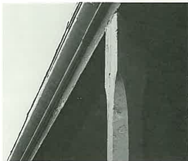
1842 gutter made by hollowing out the trunk of a tree. Mouldings have been added to give a classical profile.
