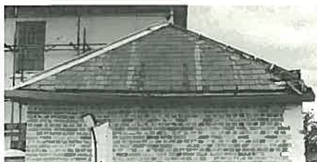
For most of the nineteenth century the traditional ridging was lead over a timber roll. In this derelict example enough detail survives for accurate restoration. (Willandra House, Ryde, Sydney. Photo: Ian Stapleton)
