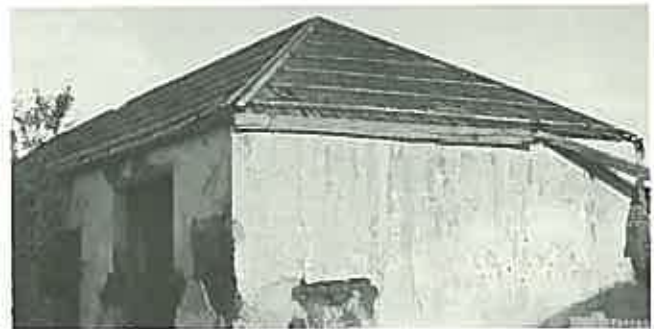
When shingled roofs failed they were often battened and sheeted with corrugated iron. (Cottage now demolished, Cleveland, Tasmania)
