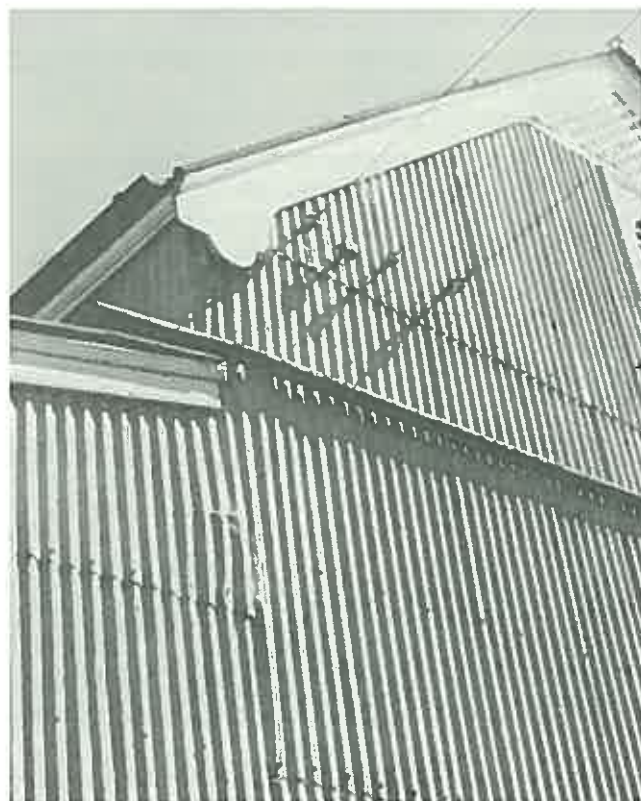
Even on farm buildings, Edwardian detail was elaborate. Here an iron barge roll and timber ovolo cap the top of the stop chamfered barge board. (Woolshed, Beggan Beggan, Harden, N.S.W.)
