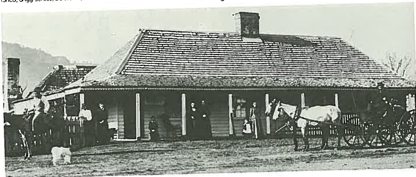
A shingle roof with iron ridging. (Kangaroo Valley Hotel, near Nowra, N.S.W. Photo in possession of D.C. Woodhill)
