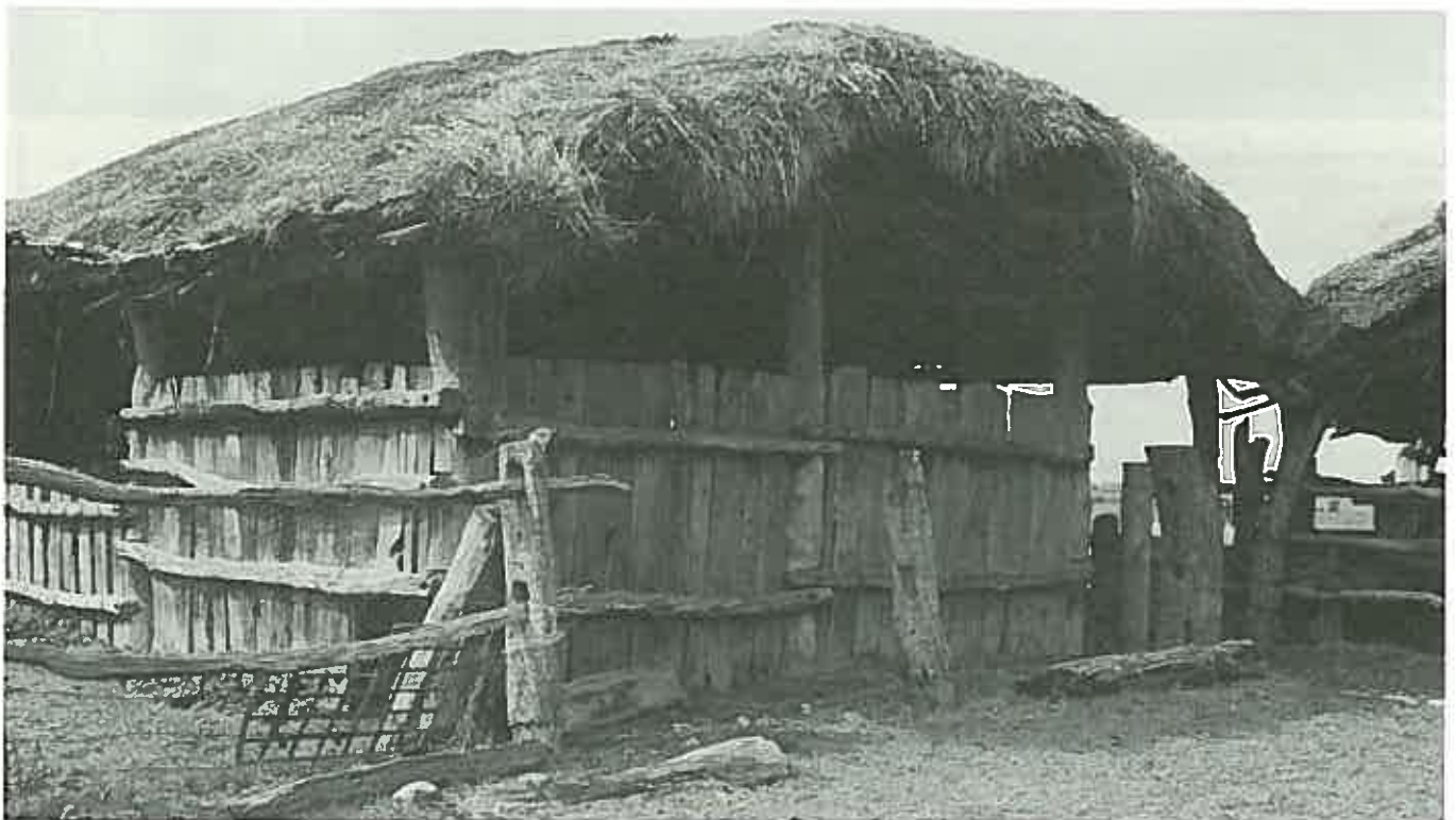
One of the earliest outstation establishments north of Adelaide. The bush pole structure is covered in straw held in place by wire netting which could be later. (Barn, Stone Hut, S.A. Photo: Stephen Gilbert)
