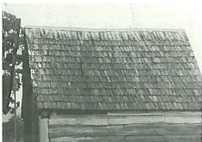
The more normal sized shingle. (Outbuilding, St Mary's, Tasmania)
