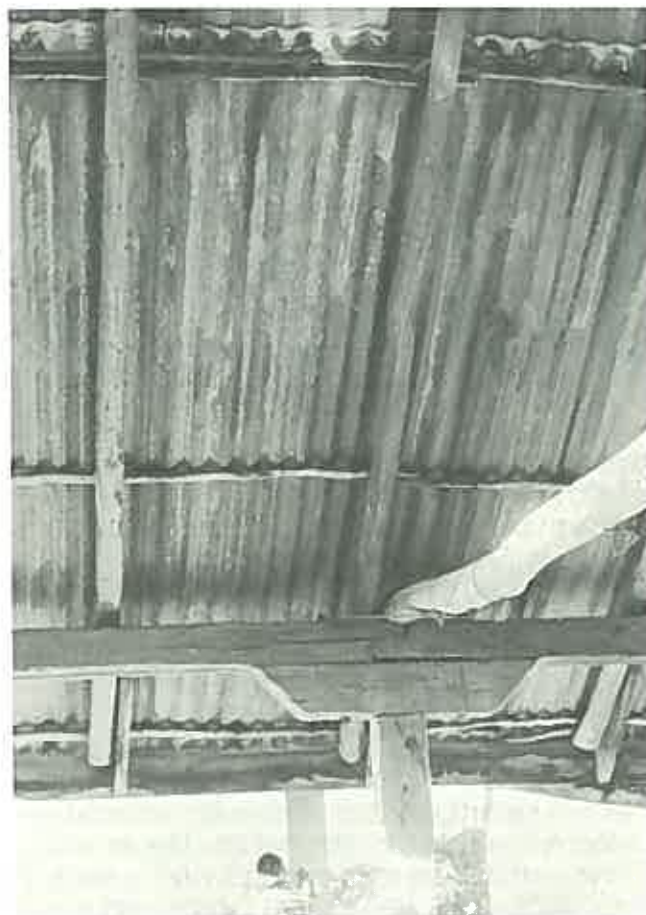
An early corrugated iron roof supported on bush pole rafters and battens. This detail would need to be carefully considered. (Chateau Tahbilk, Tahbilk, Victoria)
