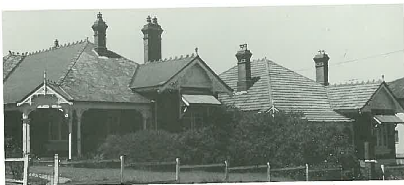
At the beginning of this century Marseilles patterned tiles were as popular as slate. In these contemporary houses one owner chose the slate with terra cotta ridging while the other, a roof completely of new clay tiles. (Houses, 471-743 Liverpool Road, Croydon, Sydney)
