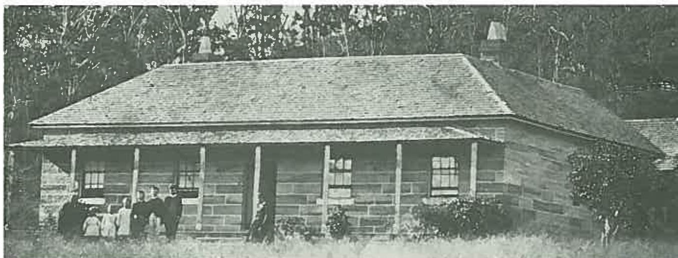
An 1850's shingle roof with woven hips. (Buxton Cottage at Glenmore, near Camden N.S.W. Photo in possession of Miss Grace Moore)
