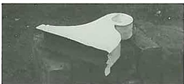
With the introduction of terra cotta tiles iron roofs were often painted tile red and plumbers made up finials to simulate terra cotta details. (Excelsior, Bathurst, N.S.W.)
