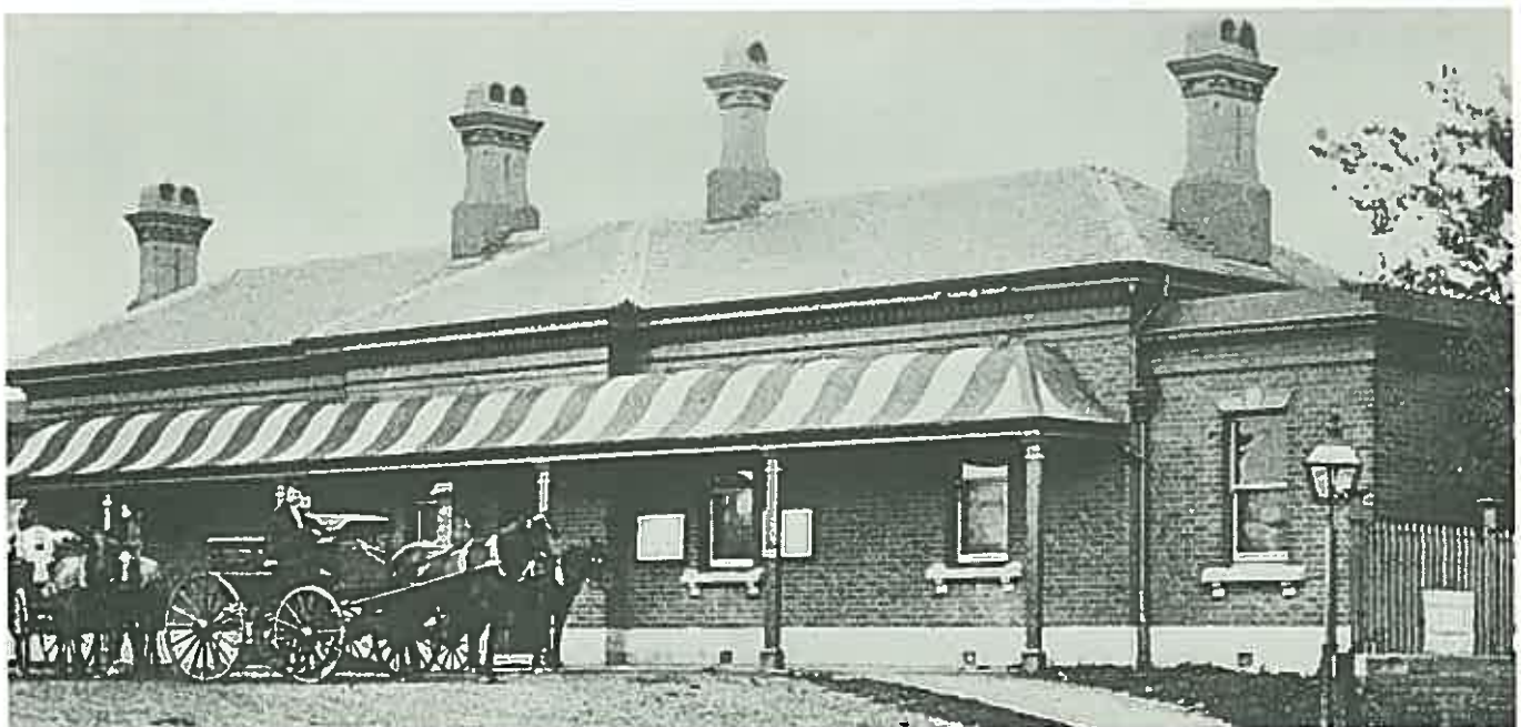
The curved verandah roof is here enlivened by the popular 19th century use of painting in stripes. (Railway Station, Richmond, N.S.W. Photo in possession of D.C. Woodhill)
