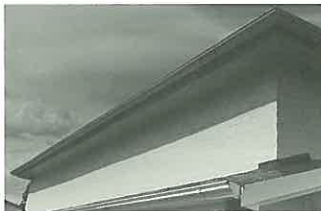
Before gutters were fitted roofs often had a generous overhang. Here ogee guttering has been fitted on extended brackets to solve this detail. (Strathmore, Nile, Tasmania)
