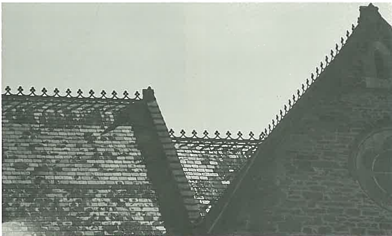
Slate roofs were sometimes enriched with cast iron cresting along the ridge. (St. George's Church, Gawler, South Australia)
