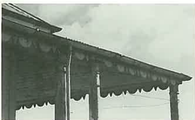
Half round galvanised guttering bracketed off a valanced veranda plate. (Throsby Park, Moss Vale, N.S.W.)
