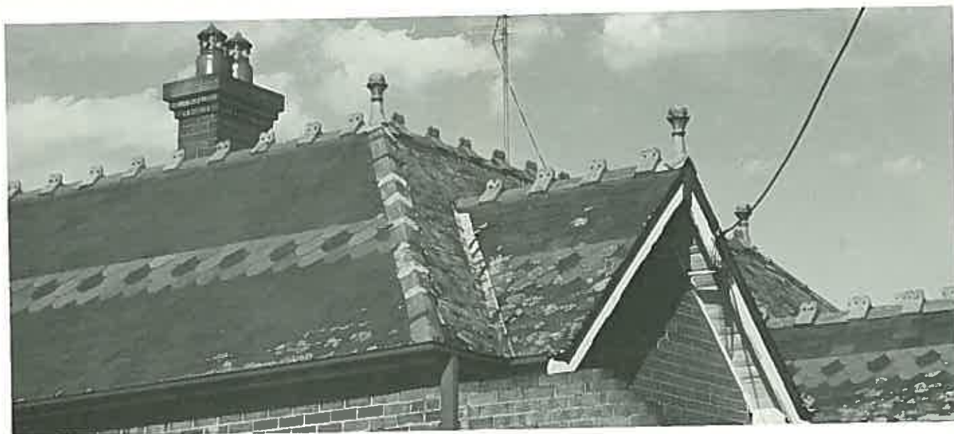
Roofs with patterned slates of different hues and shapes were popular at the end of the 19th century (Cottage, Lithgow Street, Goulburn, N.S.W.)
