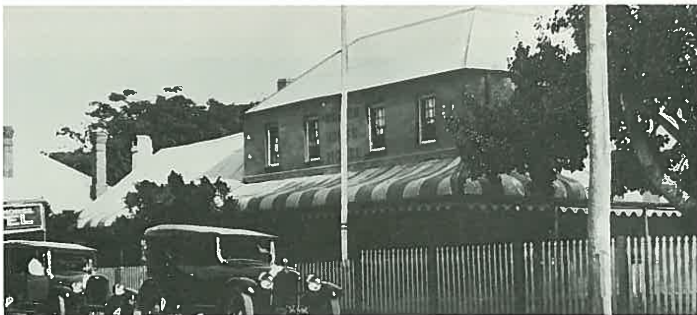
1920s photograph of the Black Horse Inn shows how it had changed with an iron roof and bullnosed roofing to the encircling verandah. (Photo in possession of J. C. Woodhill)
