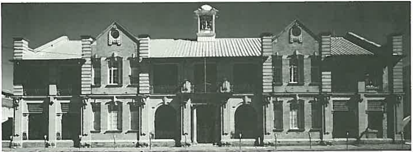
The traditional rolled zinc form continued to be popular in Queensland until well into this century; here it is carried out in galvanised iron. (Technical College, Rockhampton, 1914. Photo: Richard Stringer)
