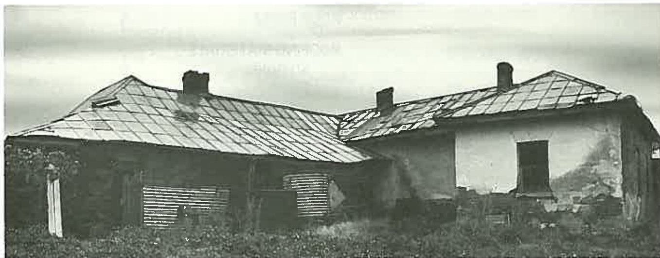
An English iron tile roof before restoration. Although in an advanced state of decay all the detail was there for exact restoration. (Cooma Cottage, Yass, N.S.W. Photo: John Morris)
