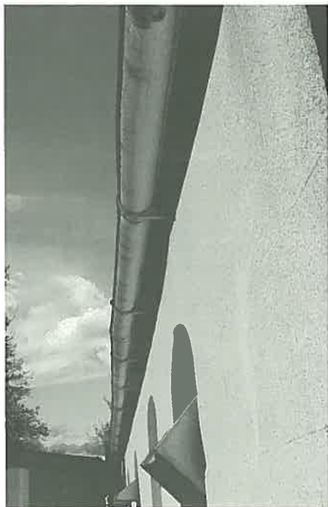
Half round galvanised gutter fixed without fascia by driving brackets directly into masonry (Vine Lodge, Exeter, N S W)
