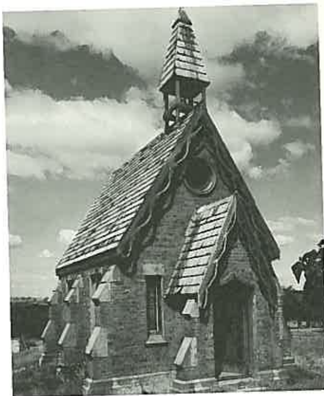
Split shingles newly restored to this picturesque building with elaborate fretted barge boards. (Chapel at Brickendon, Longford, Tasmania. Photo: Wesley Stacey)
