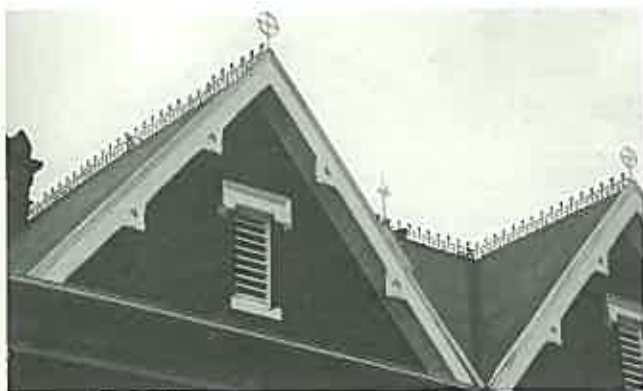
Cast iron cresting on this Edwardian iron roof. (The Presbytery, Forbes, N.S.W.)
