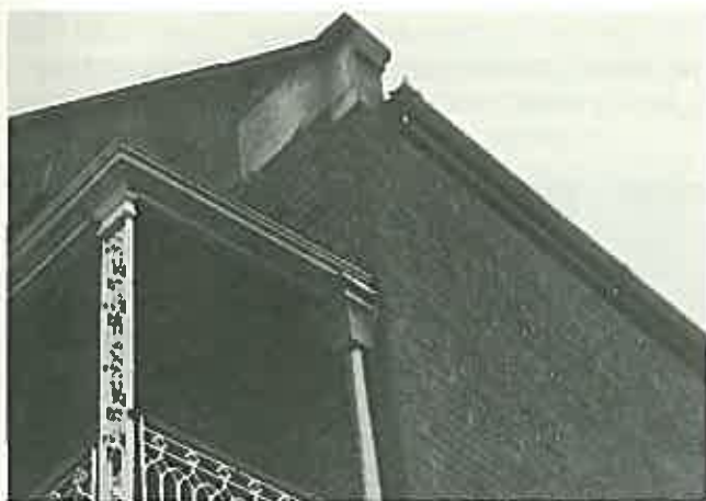
Half round cast iron gutters on the main roof, ogee galvanised gutter on the balcony.
