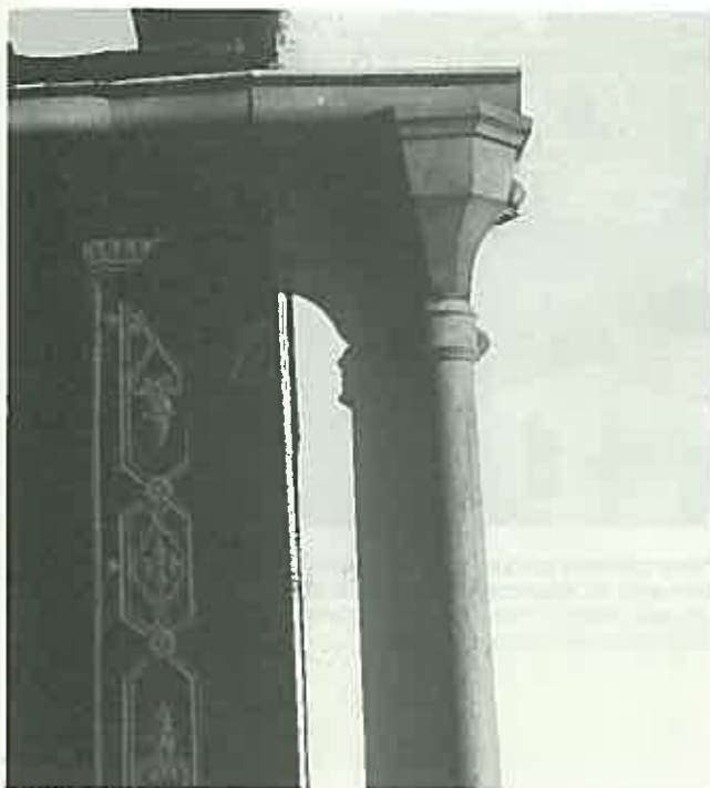
In older buildings cast iron rainwater head and downpipes often survive and if possible should be retained. (Elizabeth Farm, Parramatta, N.S.W.)
