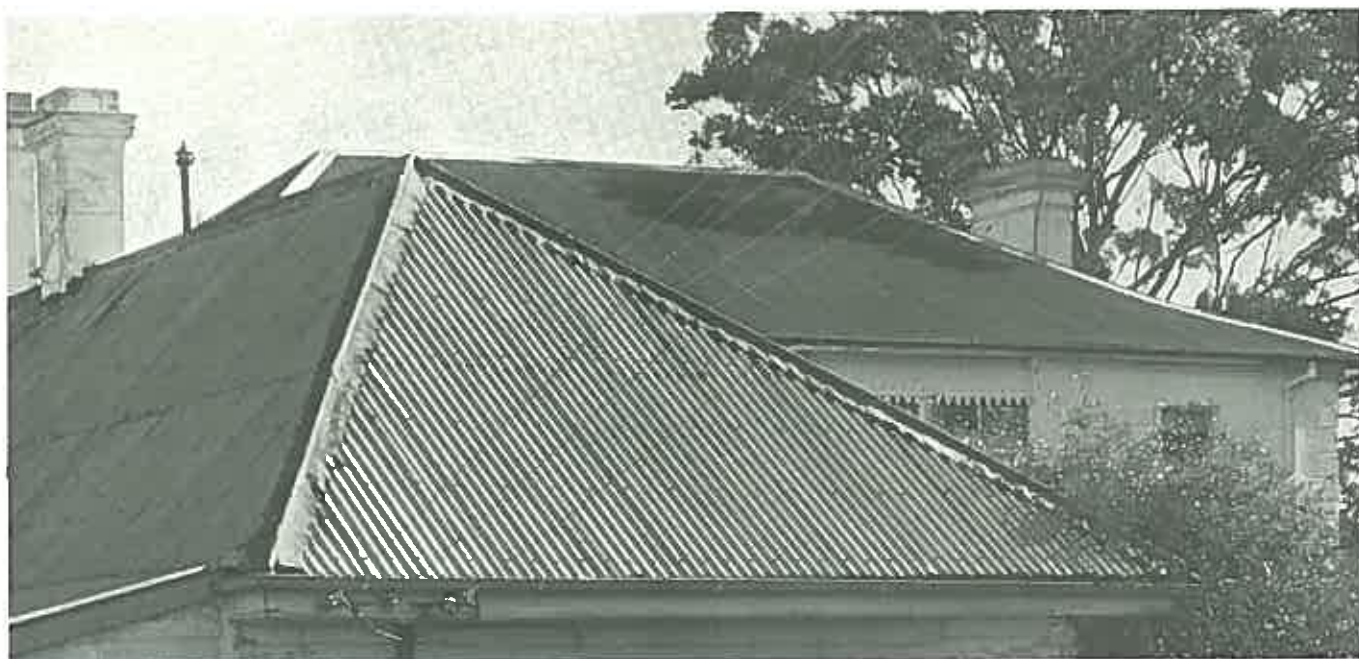
The traditional lead covered ridge roll used with corrugated iron. (Glenlee, Menangle Park, N.S.W. Restoration Architects: Fisher Lucas)
