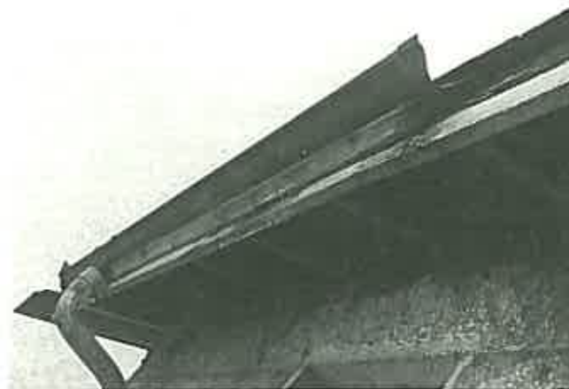
Cast iron ogee gutter with downpipe dating from last quarter of 19th century. (Cell block, Beechworth, Victoria)
