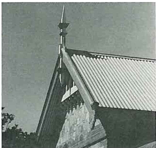
A square finial built up with applied mouldings. Such mouldings have often fallen away. Surviving fragments should be carefully noted and restored. (House, 10 Adelaide Road, Gawler, S.A.)
