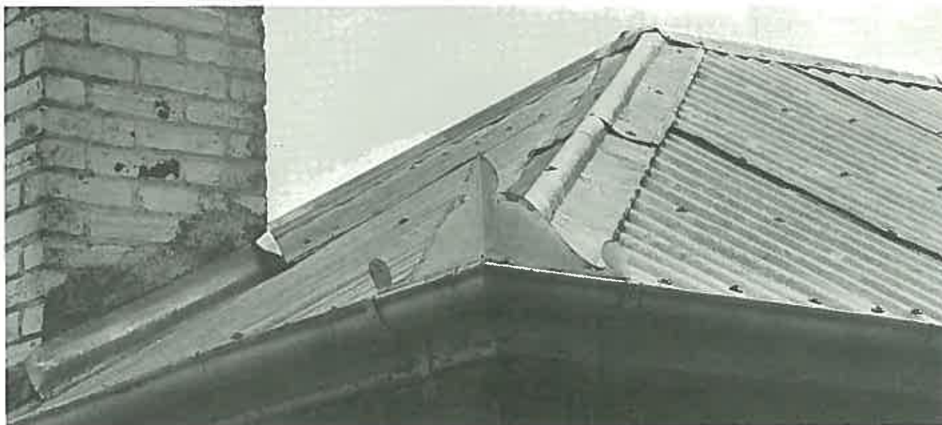
The usual iron ridging found, here with a shaped acroterion at the corners of the half round gutter. The roof is fixed by screws through lead washers. (Cottage, Ayers Street, Burra, S.A.)
