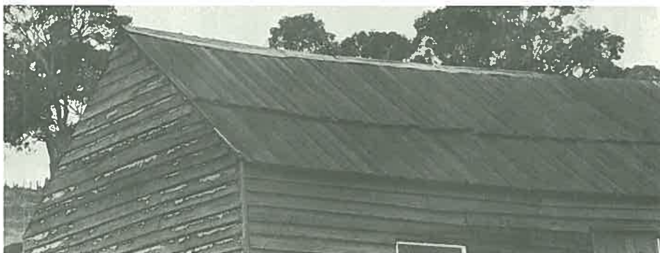
Timber roofing was also composed from sawn palings particularly for outbuildings. (Shed, Marlborough Street, Portville, Tasmania)
