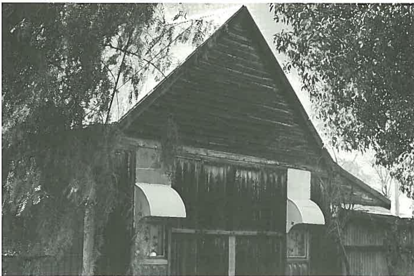
Plumbers also made up sun hoods. (House, Tambo, Queensland. Photo: National Trust of Queensland)
