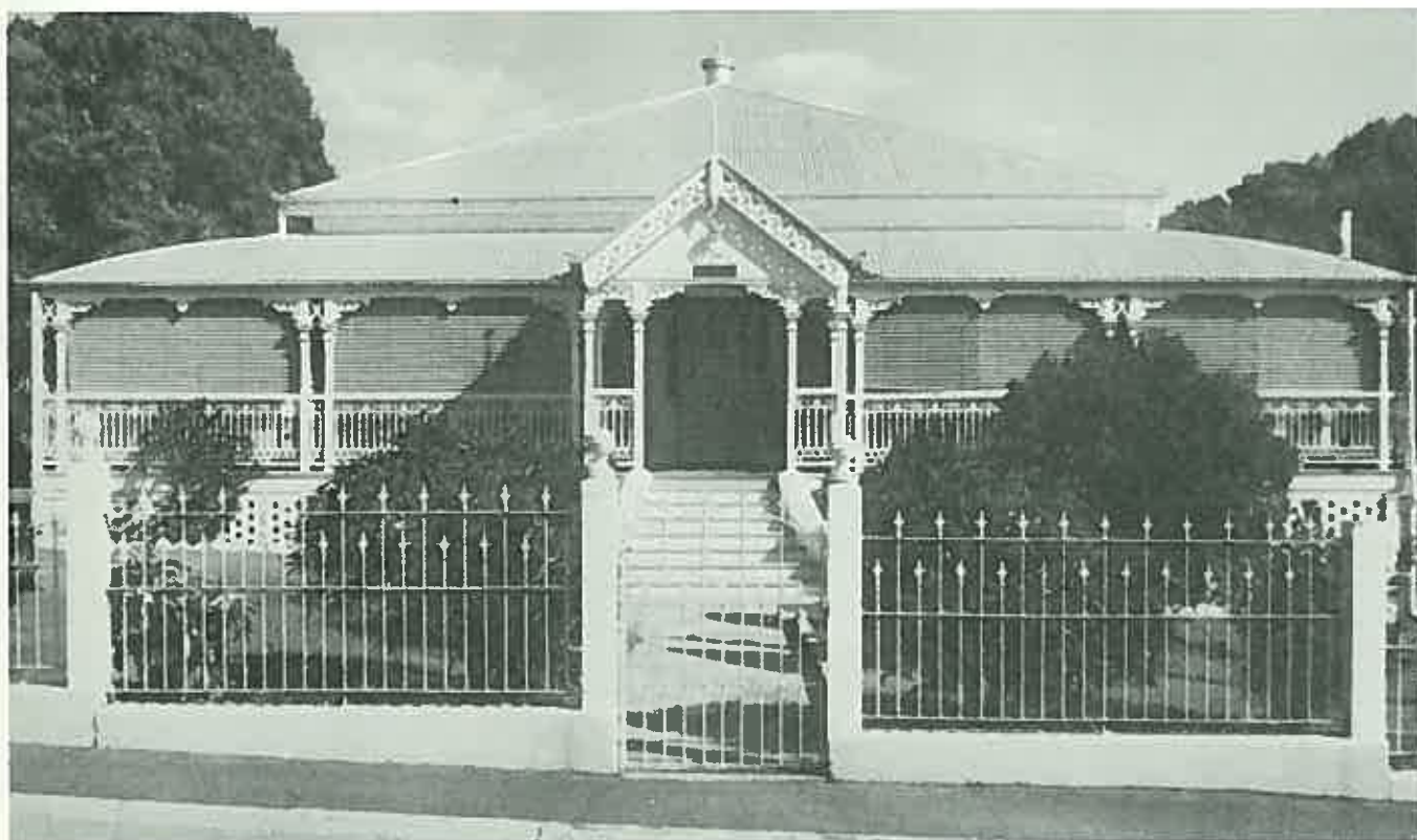
The roofs of northern houses are invariably capped with ventilators. (House, Townsville, Queensland)
