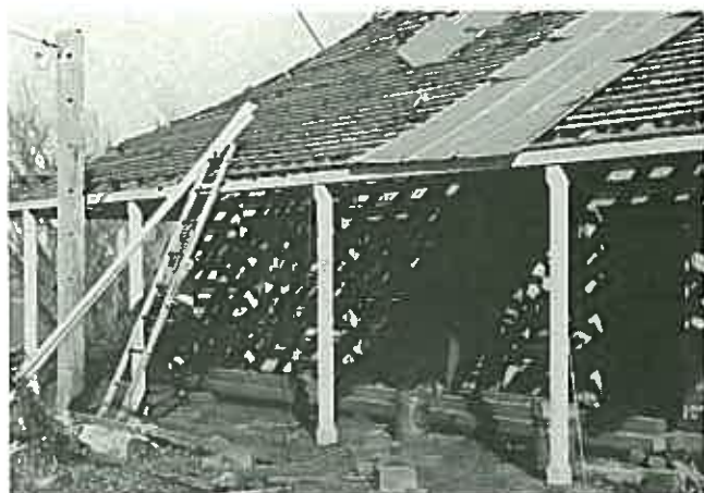
Iron tile roofing being restored. The battens of the original shingle roof survive and have been used to support the metal. (Cooma Cottage, Yass, N.S.W. Restoration Architect: Clive Lucas)
