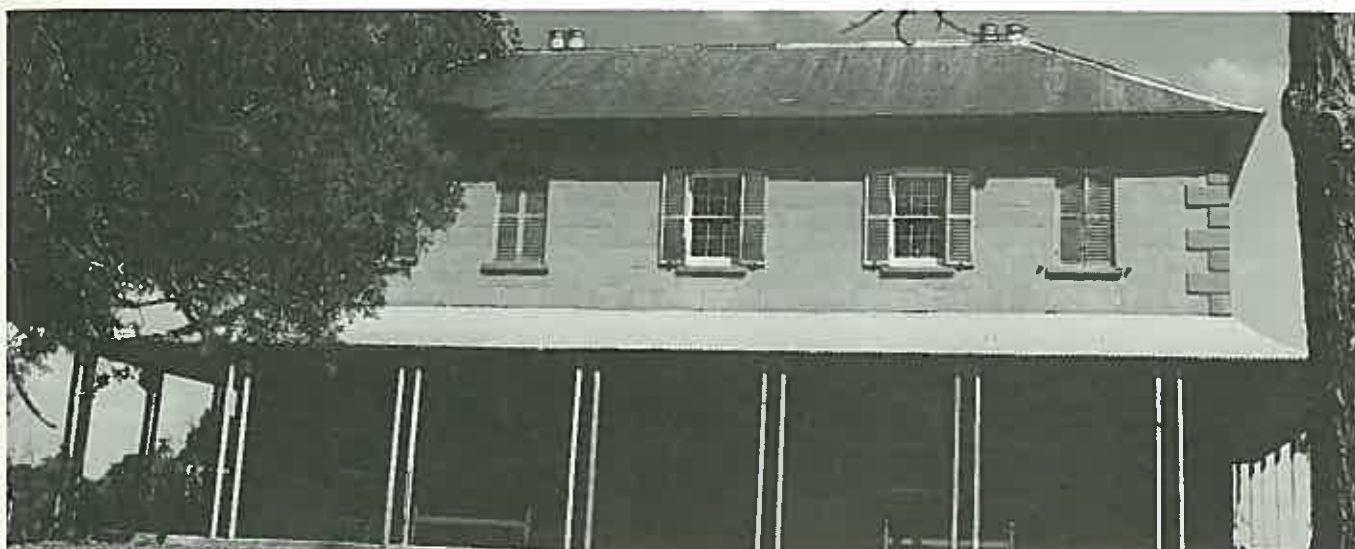
Many early Australian houses had no eaves gutters. In this example, although slates replace the original shingles, the eaves detail survives. (Rouse Hill House, near Windsor, N.S.W.)
