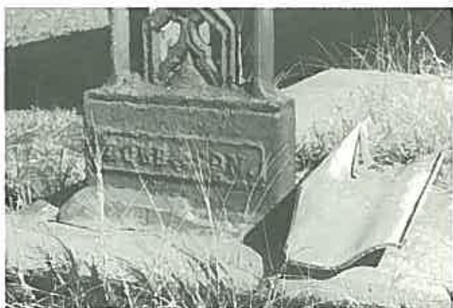
Cast iron patterned gutter probably of English manufacture and dating from first half of nineteenth century. (Elizabeth Farm, Parramatta, N S W)
