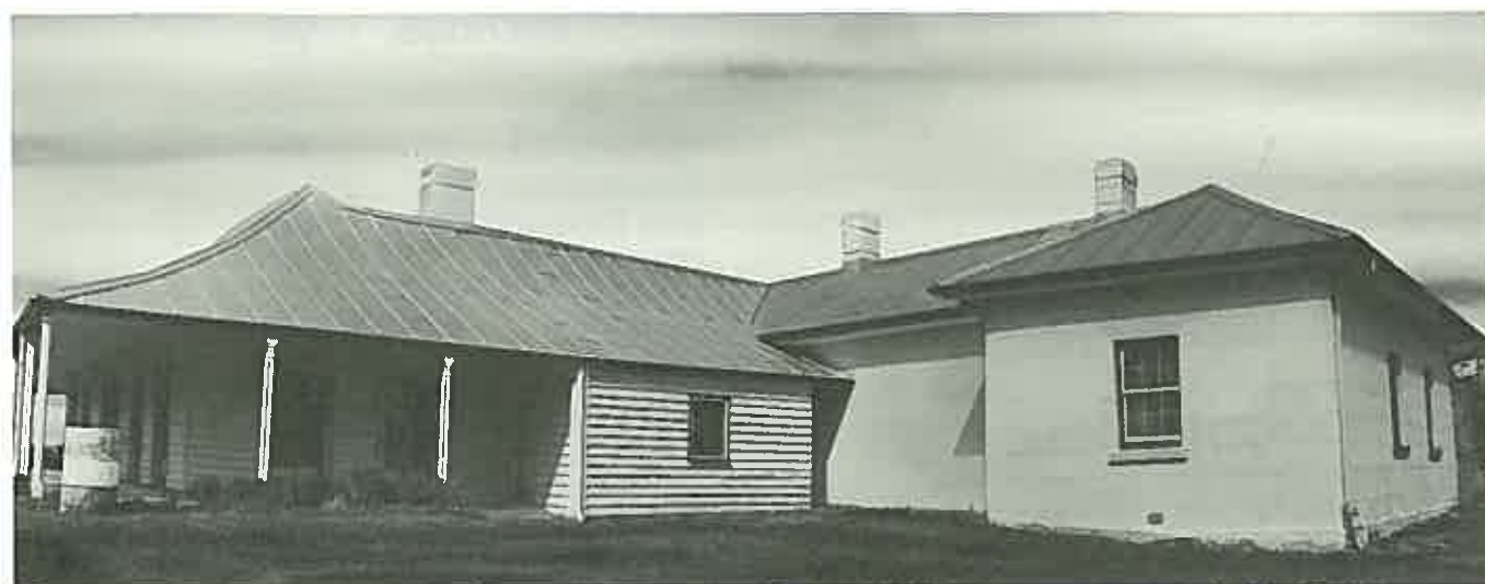
The iron tiles have been reproduced and the half round gutters reinstated. (Restoration Architect: Clive Lucas)
