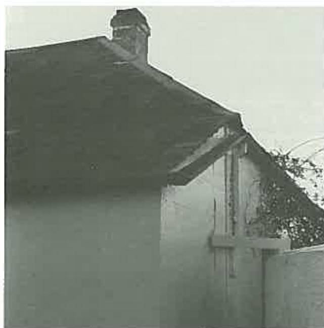
A half round gutter fixed without fascia and adjusted to suit the falls of the roofs is a surviving 19th century detail. (Horsley, Dapto, N.S.W.)
