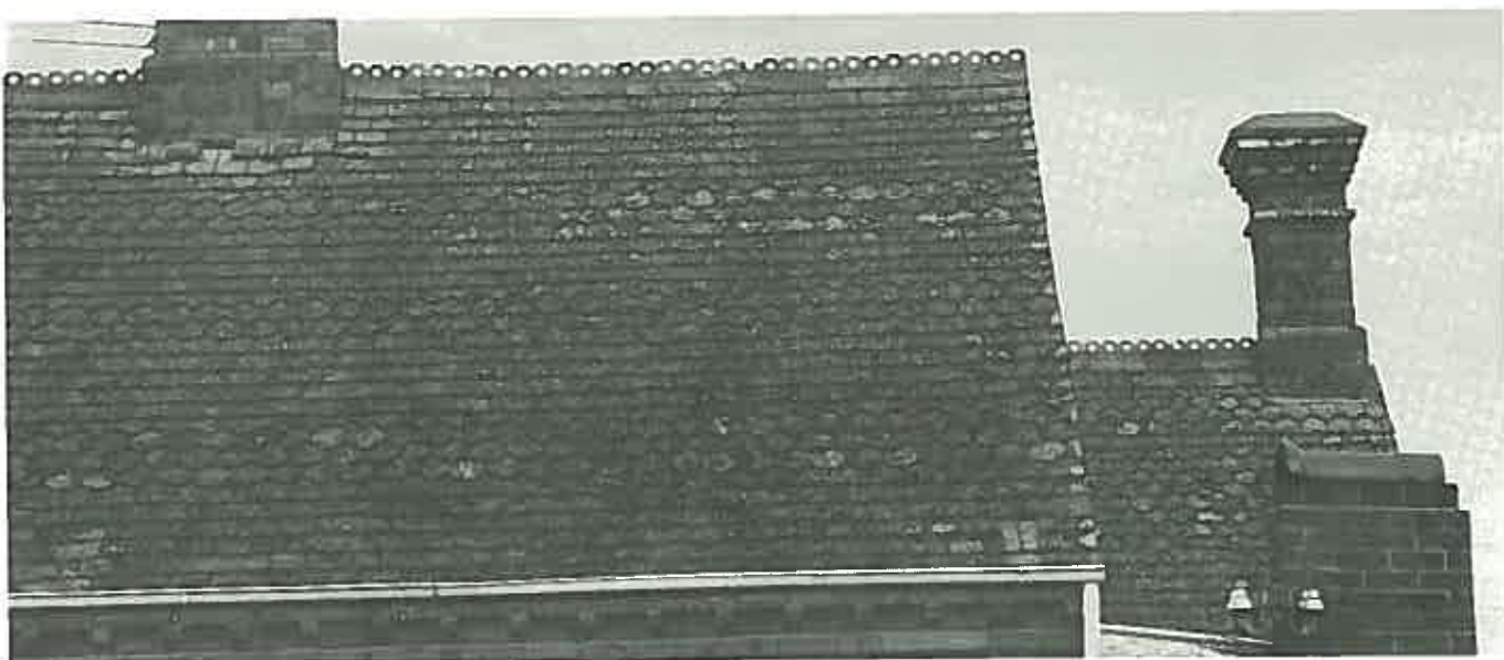
An elaborate use of flat terra cotta tiles in the 1890's (House at Gulsor's Brickworks, Goulburn, N.S.W.)
