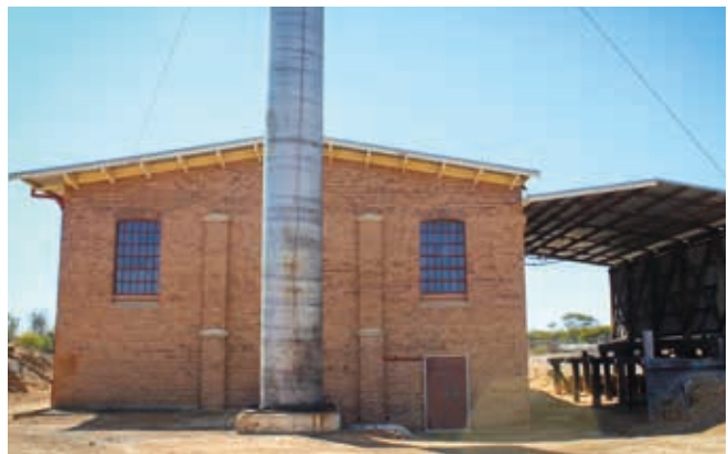
ABOVE: No 8 Pump Station. K Rippingale TOP RIGHT: Dedari resident Dusty . K Rippingale
