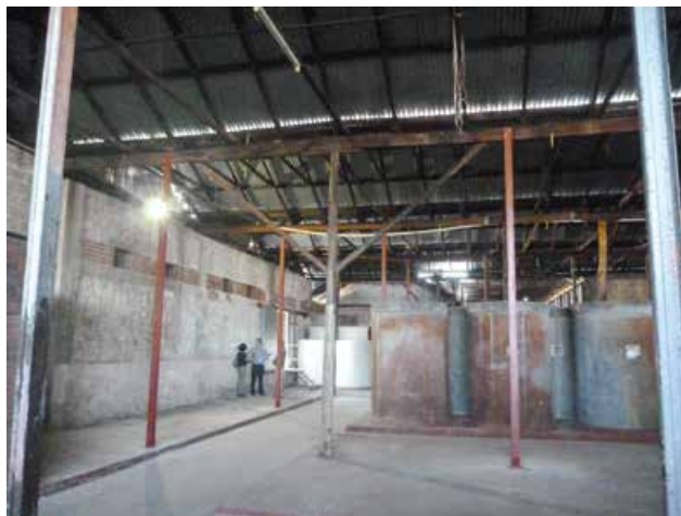
ABOVE: New security at Luisini. S Murphy
