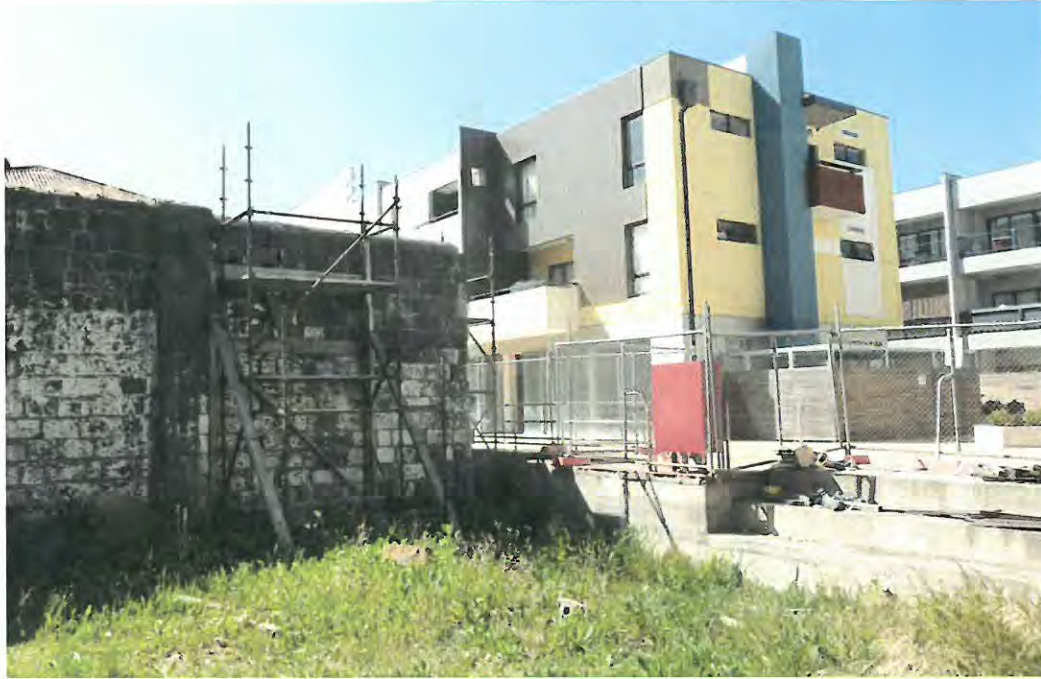
Figure 15 Recent residential development to the east of the former laundry building at Pentridge
