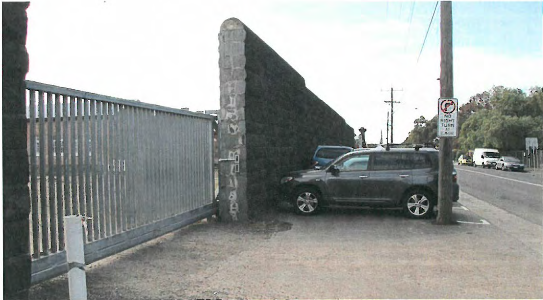
Figure 11 The existing opening at Urquhart Street
