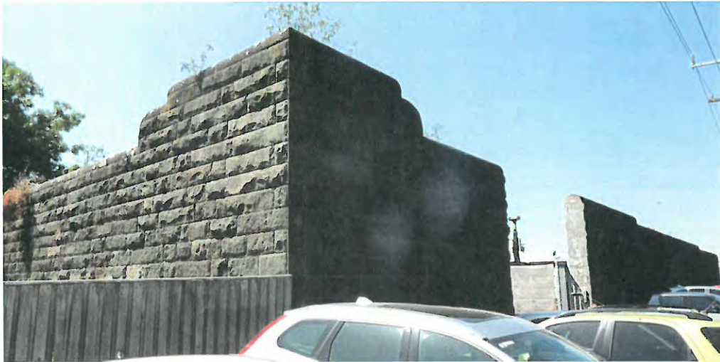
Figure 12 South-west corner of site: view from Urquhart Street
