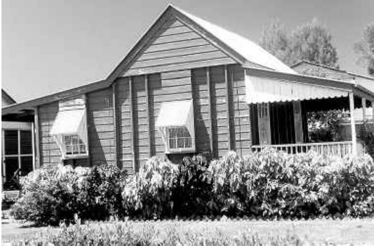
An early example of exposed framing, on the Worker's Dwelling at the National Trust Heritage Centre
