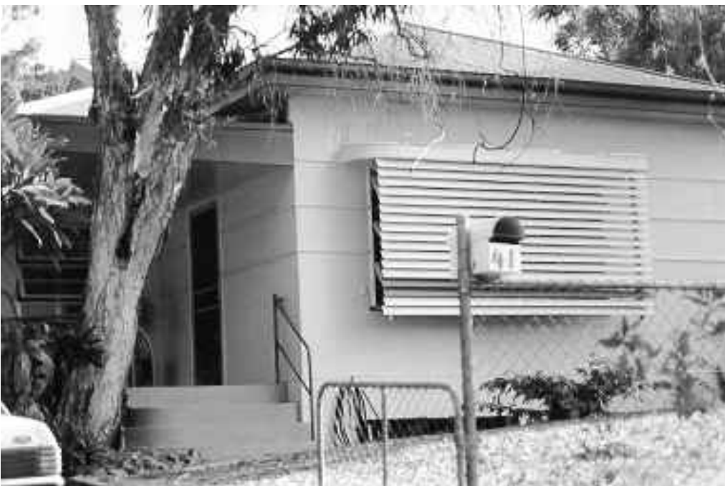
One of the earliest houses in Townsville to be sheeted externally with Fibrolite
