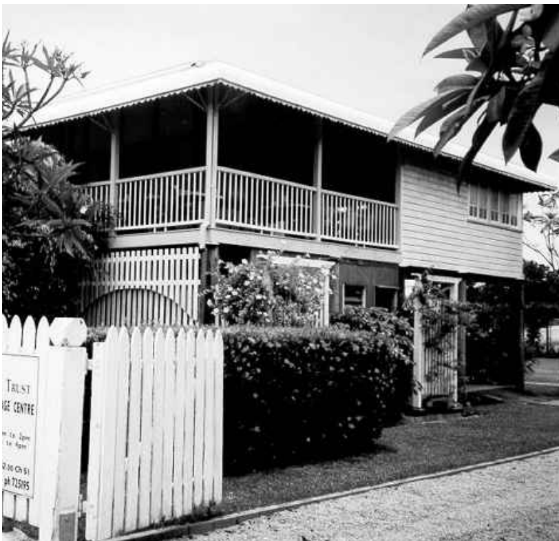
The Farmhouse at the Heritage Centre, showing chamfer boards on the rear walls
