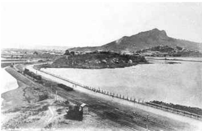
The causeway from Magazine Island to the mainland showing Pilot Hill, which was demolished to reclaim land for the sugar terminals
