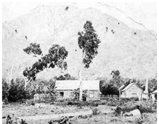
Early worker's dwelling, North Ward, about 1870.
