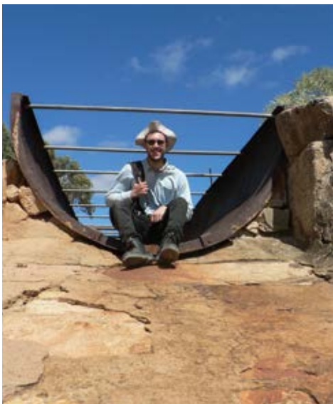
ABOVE: Timothy Mettam on the steel aqueduct at Karalee rocks. M Dossin NTWA
