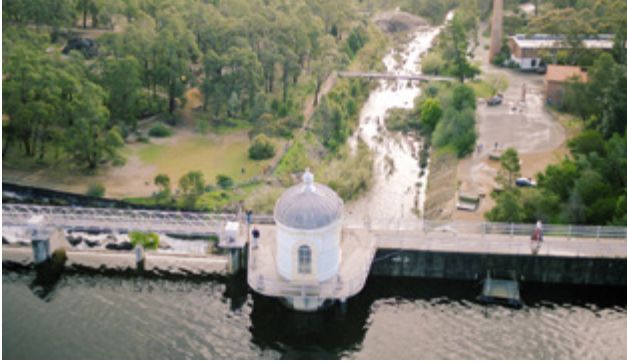
ABOVE: Mundaring Weir wall facing west with No. 1 Pump Station top right. B Birt, Water Corporation
