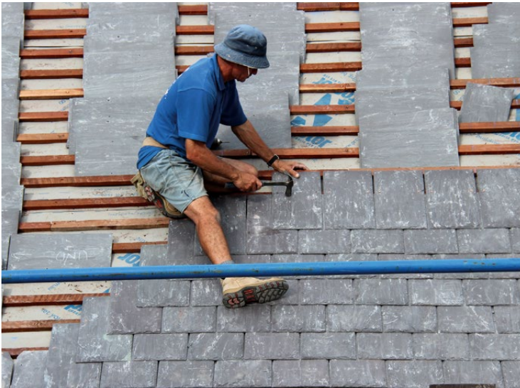
ABOVE: Slates from Wales are secured into their new positions. E Hancock.
