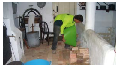
ABOVE: Staff from ABM Landscaping backfilling excavations inside Tranby. P Palmer
