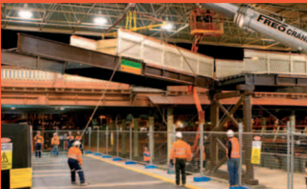
ABOVE The historic footbridge is removed by crane. Public Transport Authority
