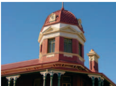
The Royal George Hotel has landmark qualities in the George Street historical precinct. National Trust (WA)
