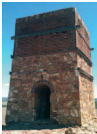
Warribanno Chimney remnants. The chimney was part of a smelting works which extracted lead mined from nearby mines in the late 1800s. A Brake/National Trust (WA)
