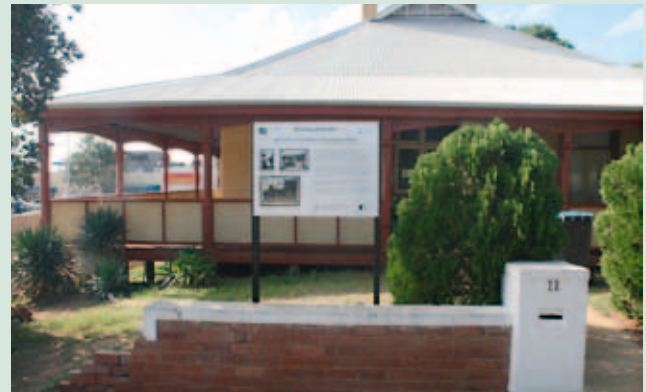
Rosella House was designed in 1912 by immigrant architect Herbert Eales in a derivative of the Arts and Craft Style. National Trust/C Stokes
