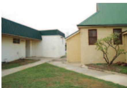
Bill Sewell Complex master plan will guide connections between the old and the new(er). Here the 1863 gaol and its 1979 version, the maximum security gaol, meet. National Trust/S Murphy.
