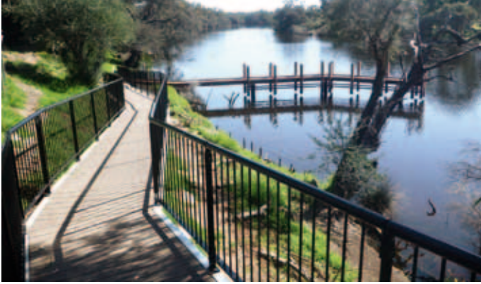
The new path and jetty at Woodbridge provide improved access to Woodbridge and the banks of the Swan River. P Palmer.
