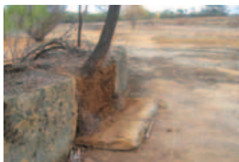
Regrowth vegetation has had an adverse impact on heritage water catchment structures at Karalee Rocks. E Hancock/National Trust (WA).
