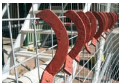
Original brackets were reinstated during works on the roof. G Pickering
