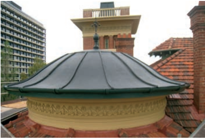
Repairs to the Old Observatory's oriel roof have been completed. G Pickering
