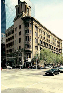
Argus building, Melbourne
