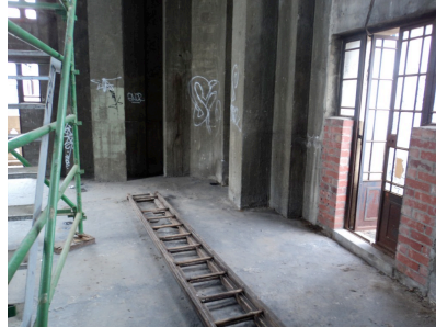
Interior of Argus building
