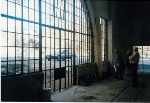
Manager of the Golden Pipeline Project, Godfrey Lowe, right, inspects the new glass doors which will help control the atmospheric conditions in No 1 Pump Station.
