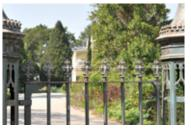
The cast iron gates located in Como Avenue were originally on Toorak Road and were erected in 1866. After subdivision and sale of land facing Toorak Road in 1911, the gates were moved to their current location, along with two cast iron lamps. Conservation work will recast missing finials to the gates, repair damage to the lamp posts and stone plinths, and clean and repaint the gates and lamps returning them to their original colour scheme and protecting them into the future.
