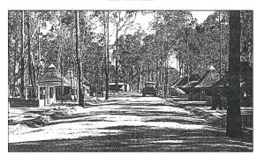
An image showing the Headquarters of the US Sixth Army at Camp Columbia is at left. The buildings were constructed using timber with asbestos cement (fibrolite) cladding.
