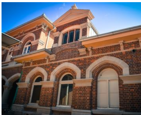
Queensland Rail, Roma Street Station Heritage Building, Stage 1 Stabilisation
