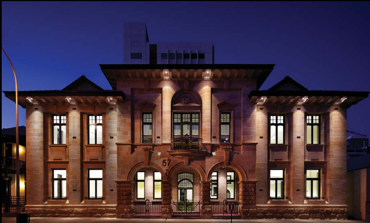
Conservation works carried out and completed by the National Trust of Australia (WA)
