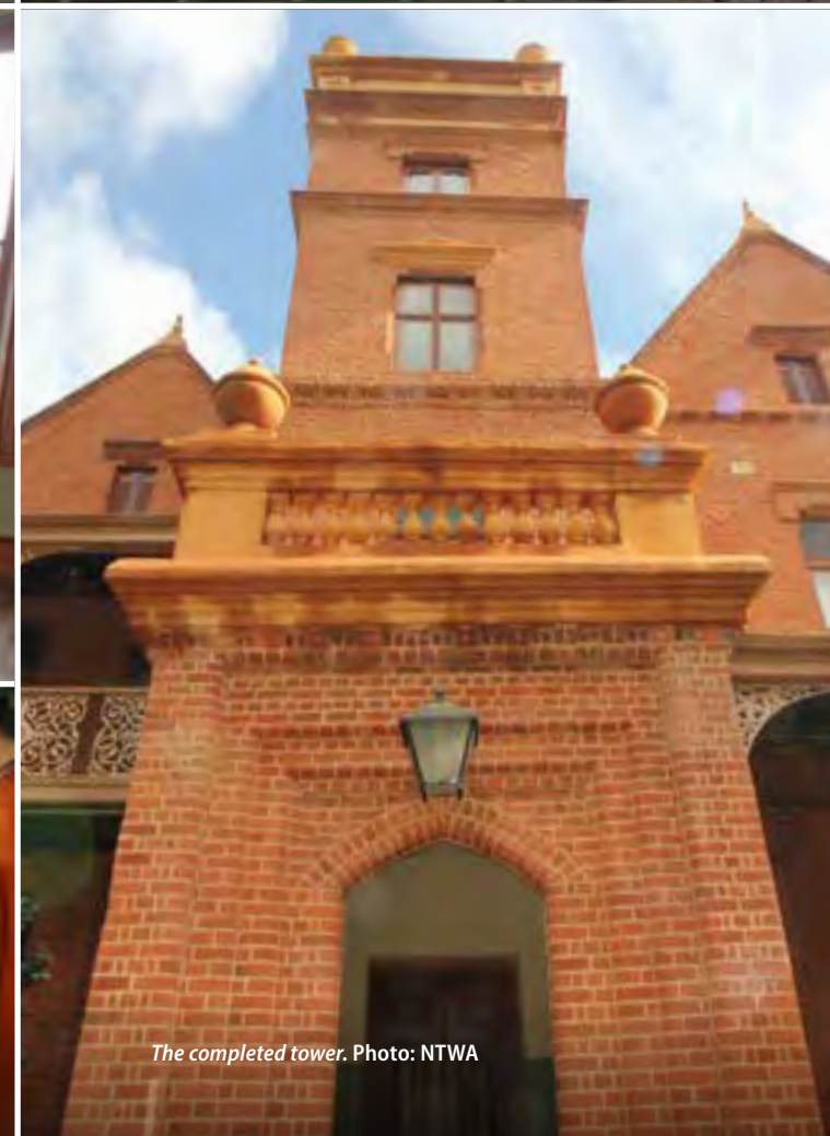
Urns and finials have been installed in pieces by crane, reinstated to replicate the original building design. Photo: NTWA
