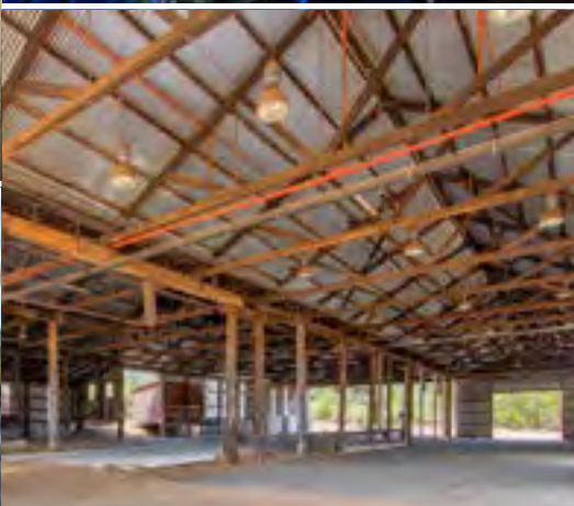
Interior with truss framework. Photo: NTWA
