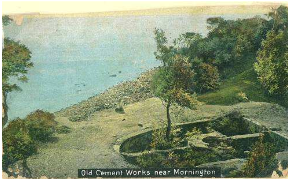
Figure 12: Old Cement Works near Mornington, post card c 1909
