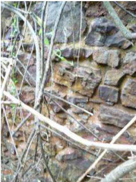
Figure 32: Internal stonework of rectangular tank
