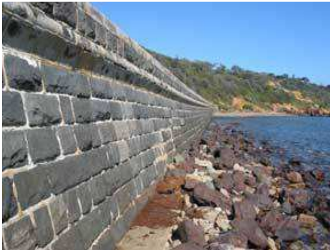
Figure 17: Looking south along sea wall
