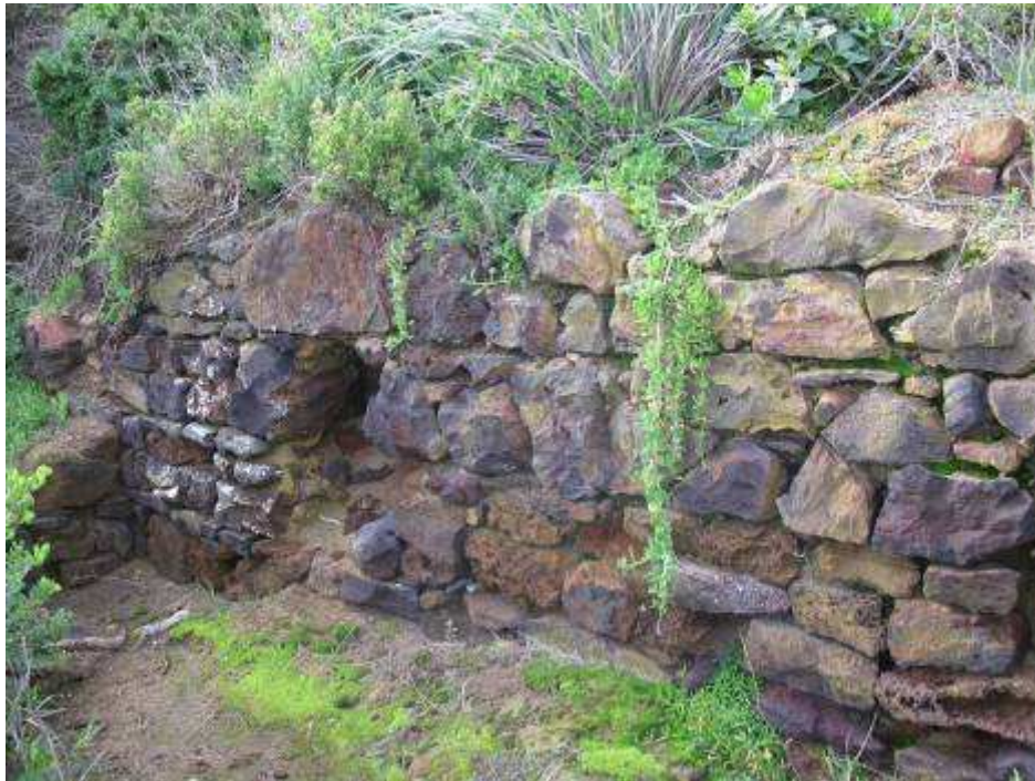
Figure 25: Retaining wall south of large kiln.
