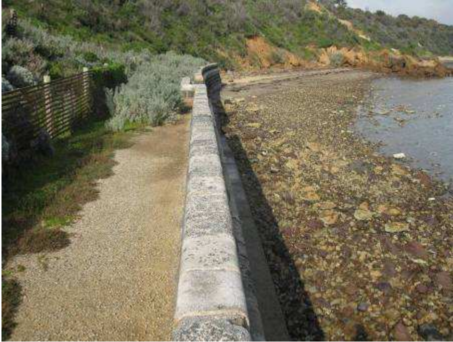
Figure 18: Sea wall looking south, note revegetation area on left and mix of Baxter sandstone and limestone on the rocky shore
