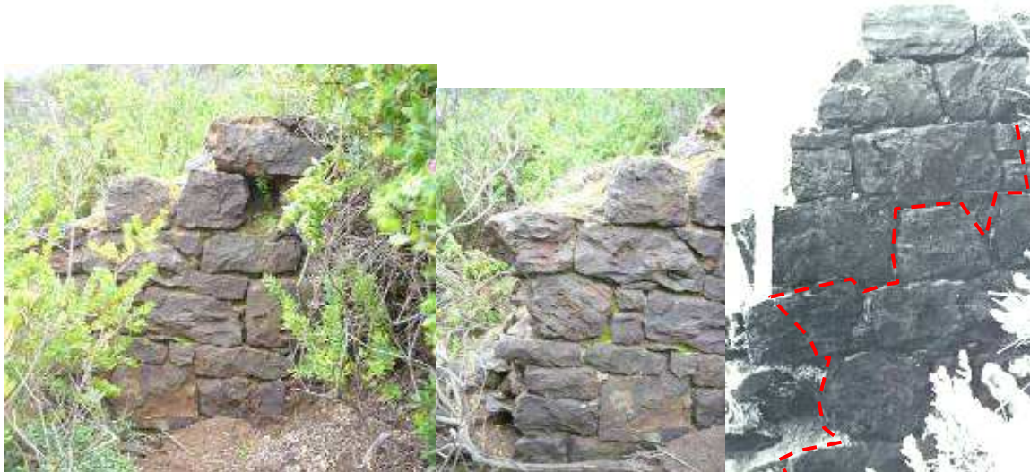
Figure 23: Outer surface of southern wall of large kiln, showing line of surviving stone on Culican's c1970 photograph.
