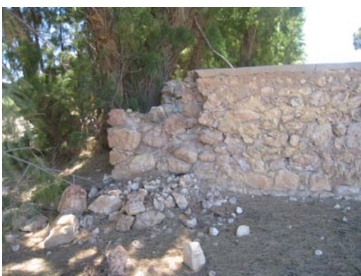
Collapsed wall, Central Greenough due to water penetration of cap course. Funding to facilitate a minor repair would have prevented this loss.
