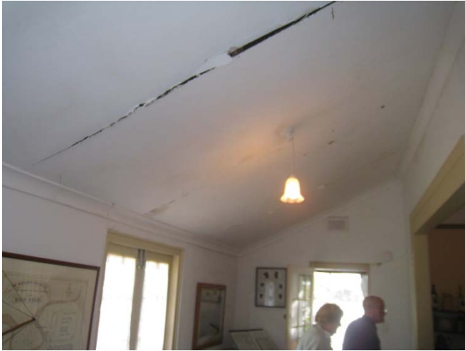
Ceiling delamination caused by roof leaks, Peninsula Farm, Maylands
