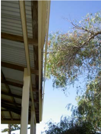
Replacement gutters rusted through due to lack of maintenance funding
