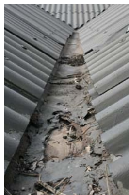
Rusted box gutter, Bill Sewell Centre, Geraldton
