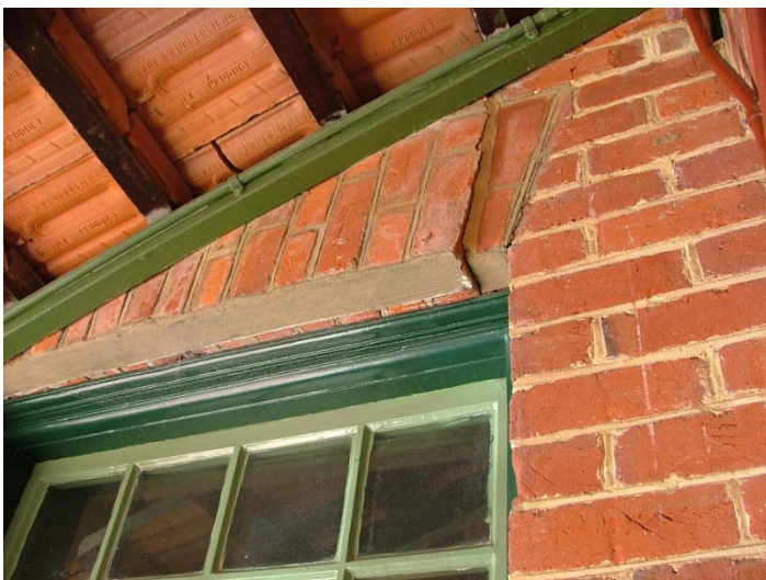
Sideways expansion of rusting lintel, Old Observatory, West Perth
