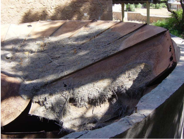
Collapsed well lid, Central Greenough
