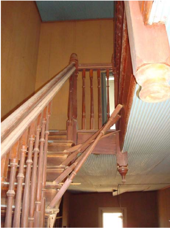
Temperature extremes can cause woodwork to dry, shrink and lose integrity. Staircase – Masonic Lodge, Cue
