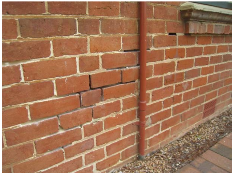
Fretting brickwork and mortar loss, Old Observatory, West Perth
