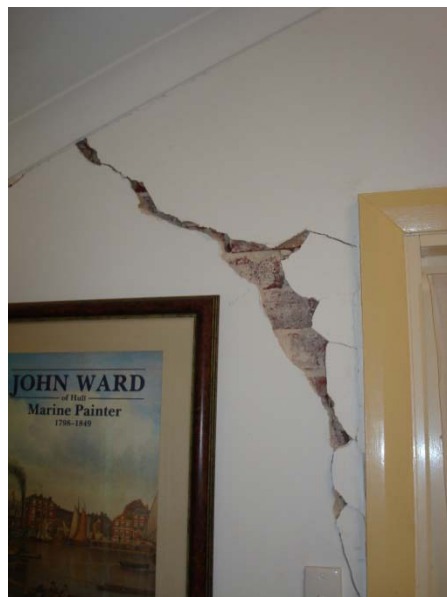
Structural cracks at Peninsula Farm due to inadequate foundations and periodic wet/dry cycles
