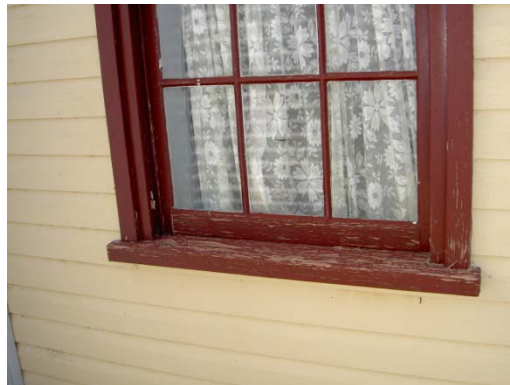
Repainting of window frame required
