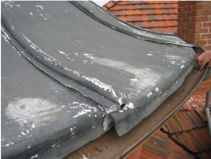
Specialist leadwork and wrought iron guttering, Old Observatory, West Perth
