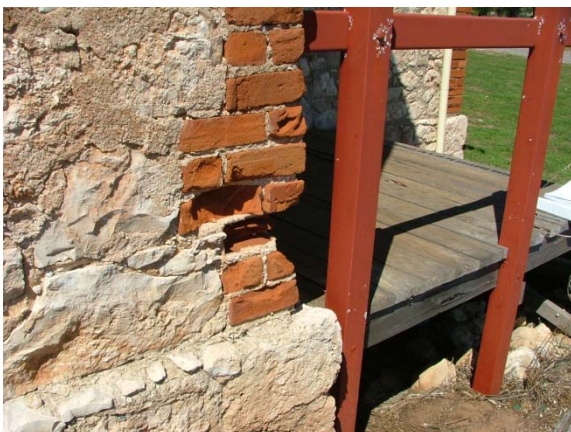
Soft brick can deteriorate quickly if associated maintenance is neglected.
