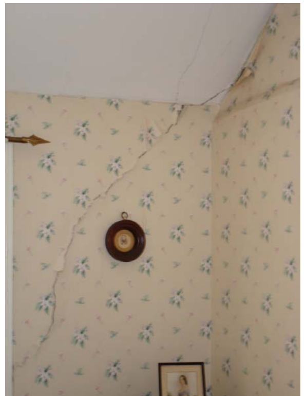
Structural cracking in part due to seismic activity and changes in soil moisture levels, Old Farm Strawberry Hill.
