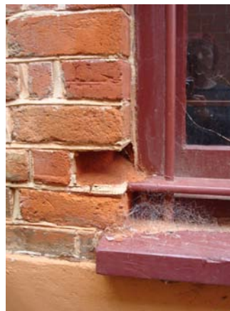
Fretting Bricks due to use of concrete mortar, York Courthouse Complex
