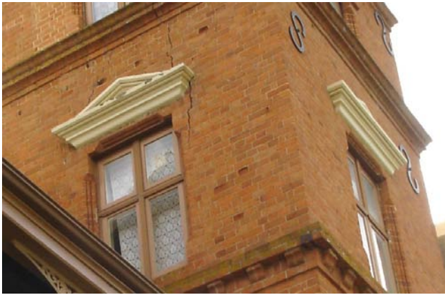
Cracks in tower at Woodbridge due to expansion of rusting lintels
