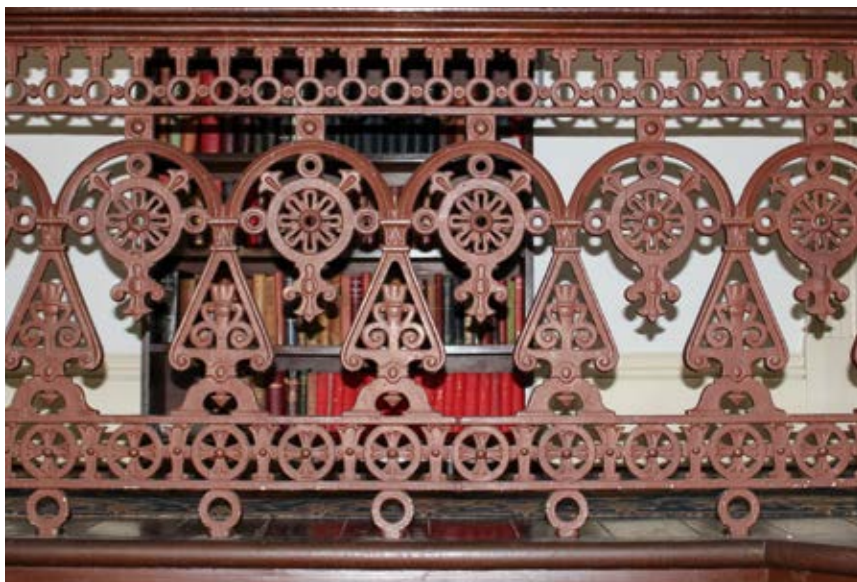
ABOVE: Cast iron panels at Woodbridge. NTWA
