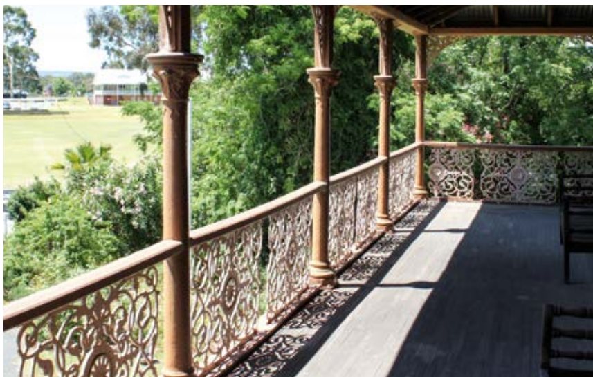
ABOVE: Compliant verandahs at Woodbridge will provide visitor access. NTWA
