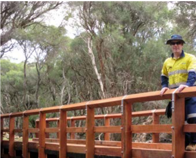
ABOVE: Peter McCleery on the completed railway bridge
