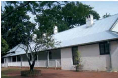
The new galvanised iron at Peninsula Farm (Tranby) provides improved protection for the building structure. E Hancock.
