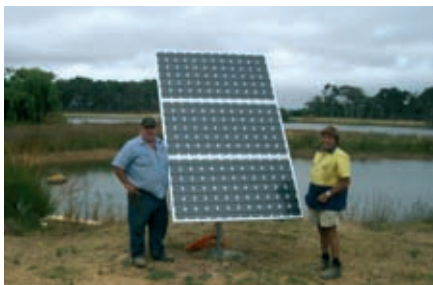
Solar panels keep the water flowing in Parkwater's entrance dam and water feature. L to r: Rob John and Gary Fletcher installation contractors. A Briggs.
