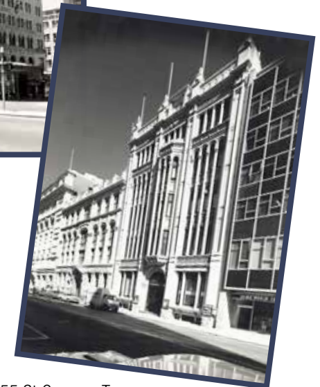
ABOVE CML Building, 55 St Georges Tce, Demolished (photo, National Trust)
