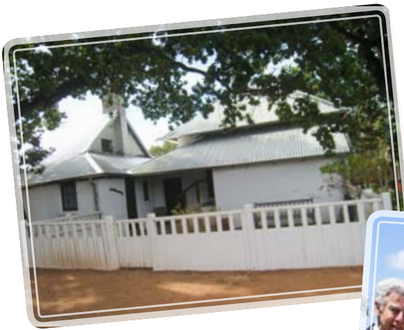
Tranby now sits dry under the cover of a new roof of short sheet galvanised iron. E Hancock, National Trust
