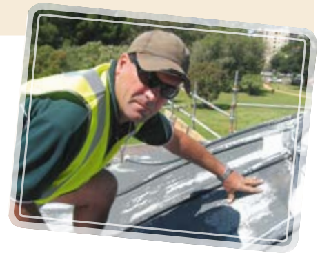
Contractor Peter Eldridge commences repairs to the oriel roof at the Old Observatory. G Pickering, National Trust
