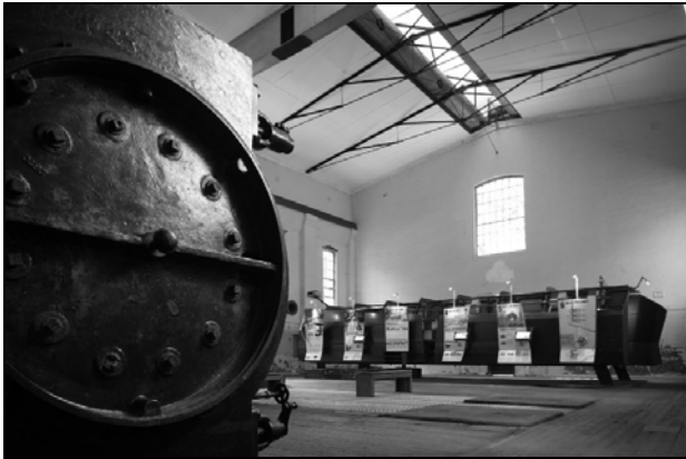
Award winning interactive interpretation at No 1 Pump Station, Mundaring Weir. Photo: R Firth
