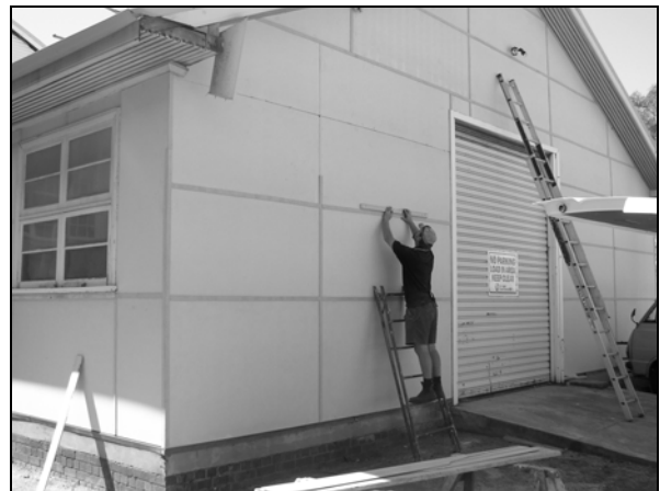
Conservation work at the Artillery Drill Hall. Photo: Kelly Rippingale
