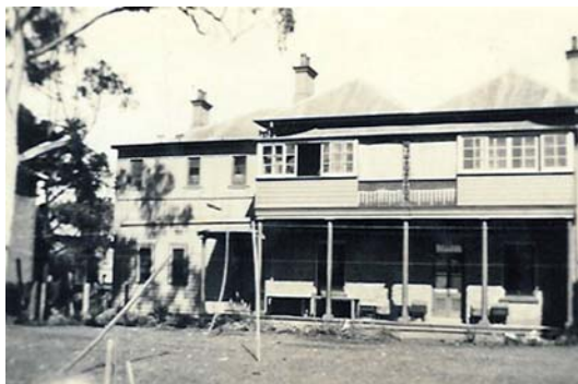
The rear of Brough House as a school boarding house 1919
